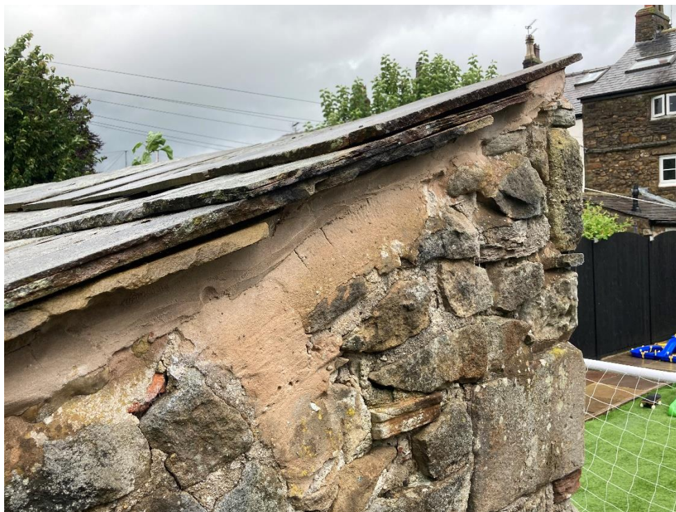
Photograph 2- View of gaps under roof slates
