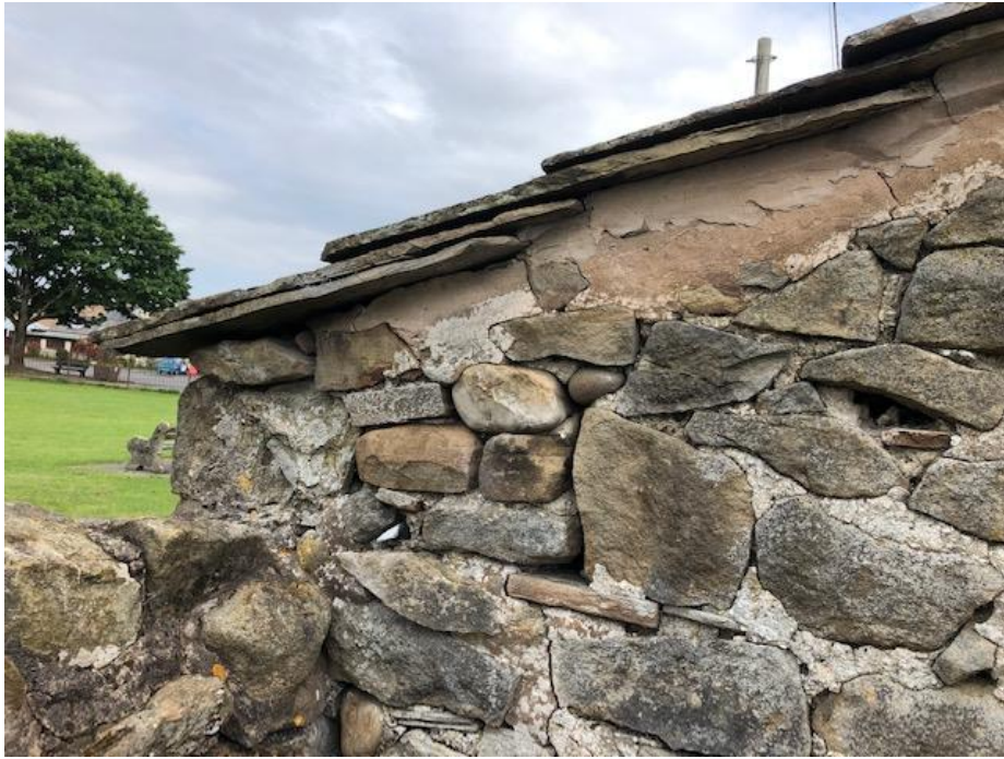
Photograph No 3: Side Elevation showing some dry verge pointing.
