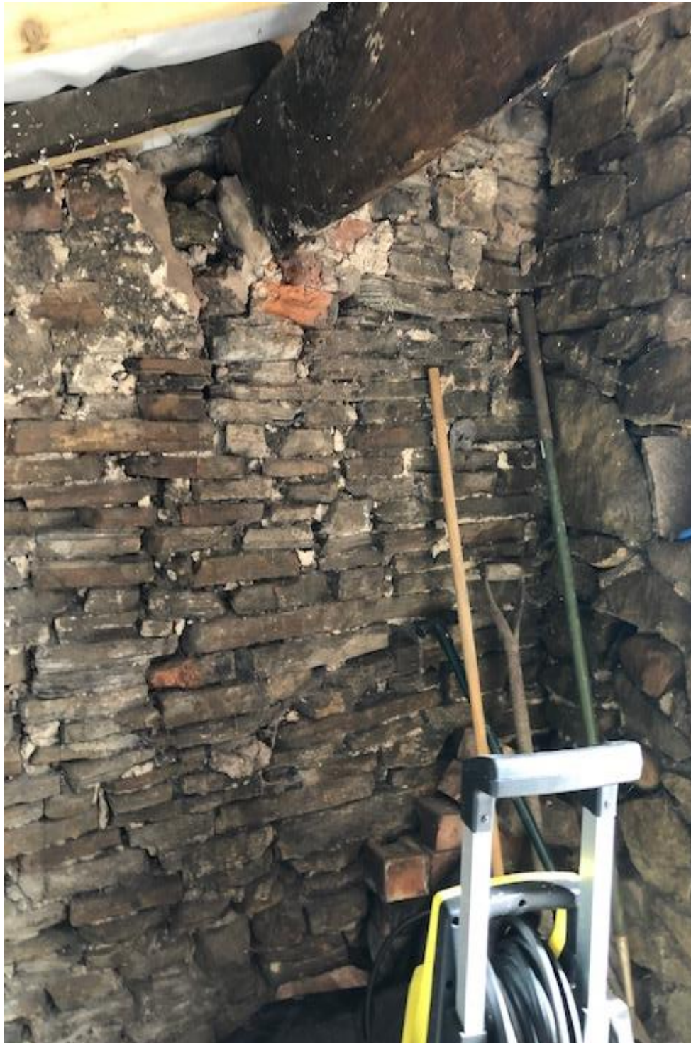
Photograph No 15: Single Skin of stonework with daylight visible supporting a structural beam. No padstone support under the beam to dissipate the weight of the beam evenly this has resulted in a structural crack which is clearly visible. Wall again is not tied into the main external structural wall.
