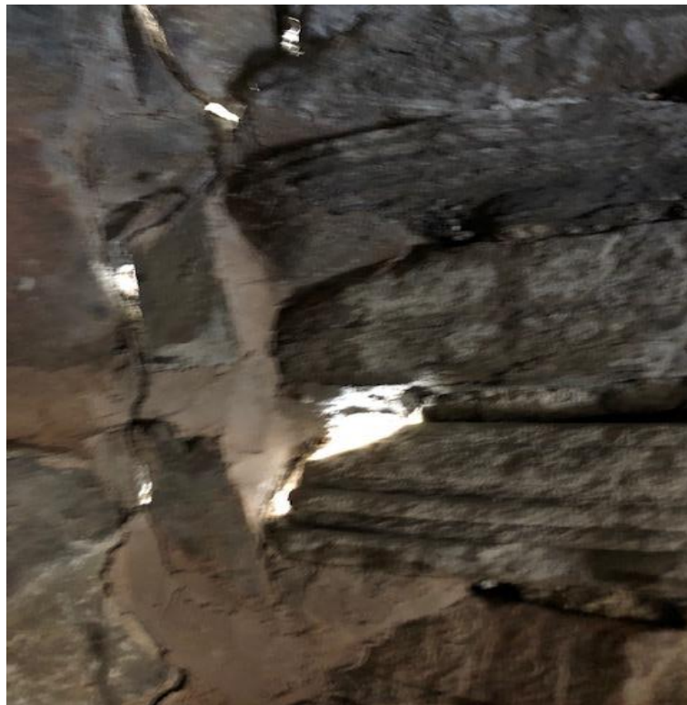
Photograph No 12: External Wall with day light visible.
