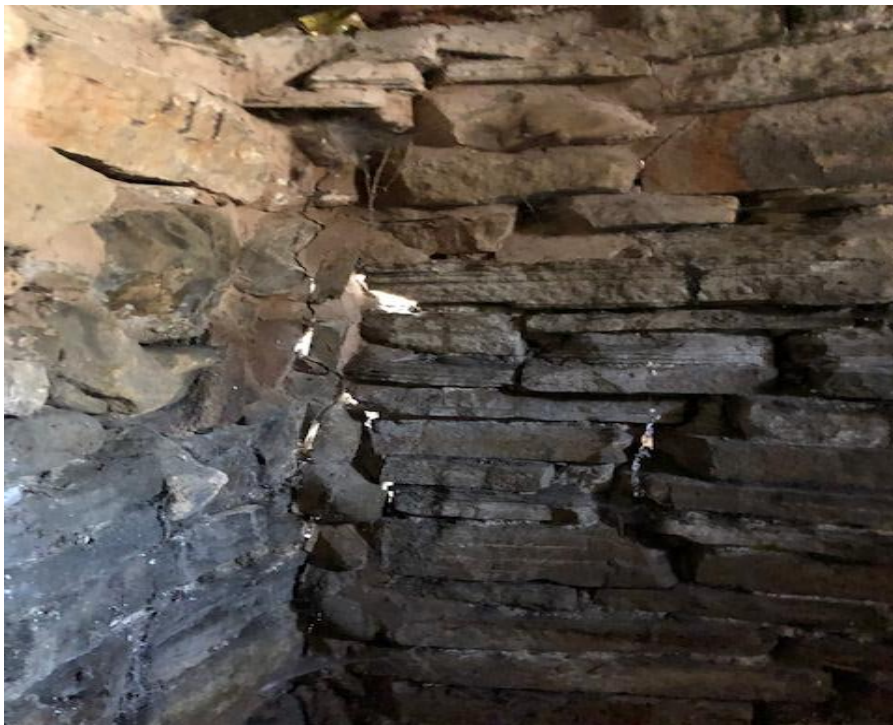
Photograph No 10: Mortar shrinkage crack plus holes within the wall construction.
