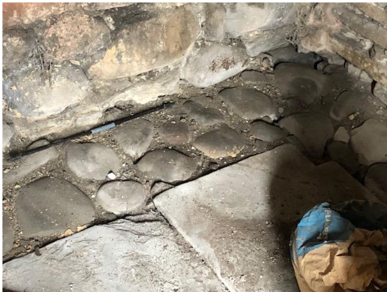
Photograph No 8: Larger Unit with “Yorkstone” slabs and river boulders as floor finish
