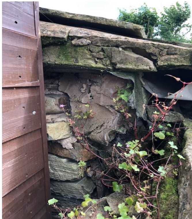
Photograph No 14: External wall stonework is free standing with no structural ties.
