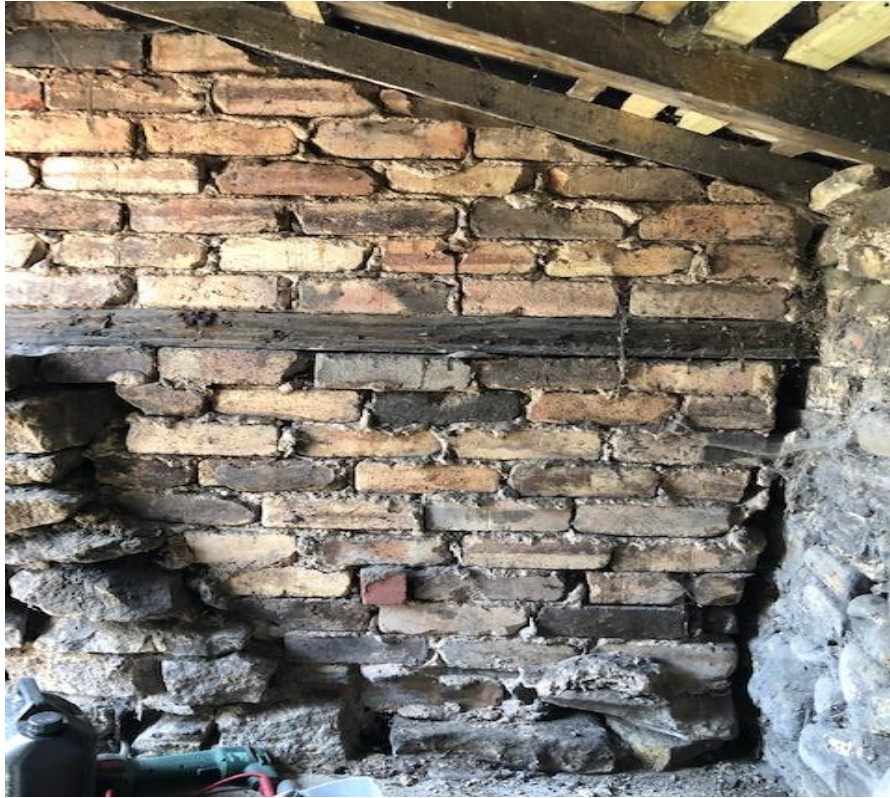
Photograph No 9: Sub-division Internal Wall showing various stages of construction. There is no structural tie into the rafter and external wall.
