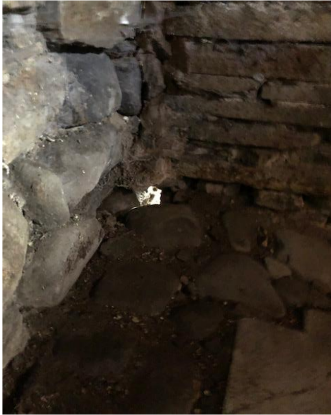
Photograph No 13: External Wall possibly built directly off floor the finish.
