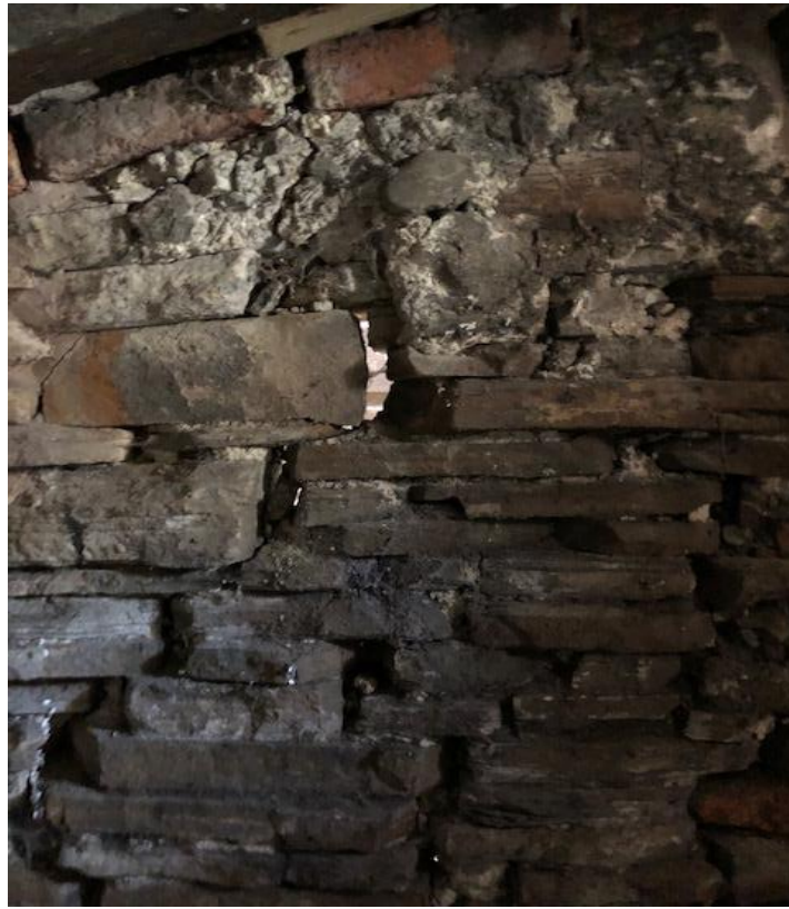
Photograph No 11: External Wall with vertical structural crack evident
