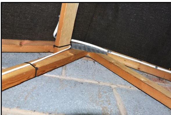
View of roof garage roof void (lhs) and main house roof void (rhs) showing bitumastic roof liner, block and brick walls and timber truss supports
