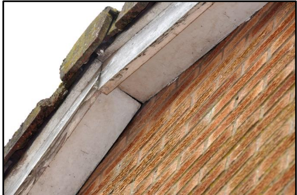
Example of gaps associated with roof corners (lhs) and gable soffits (rhs)
