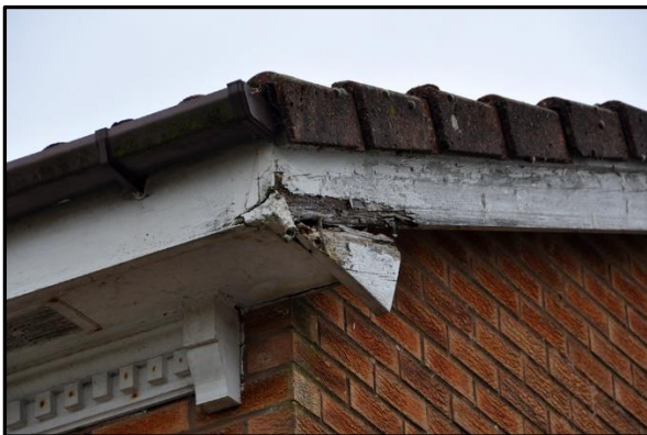
Example of gaps associated with roof corners (lhs) and gable soffits (rhs)
