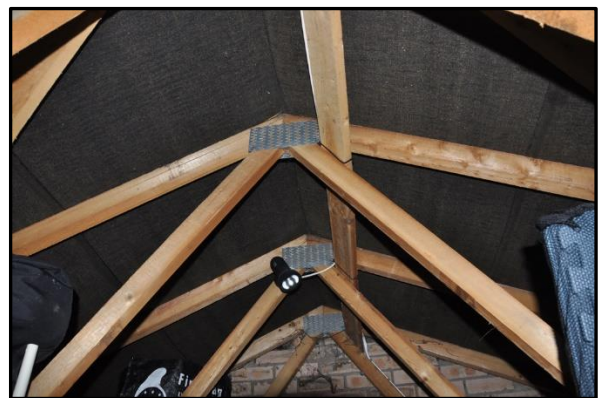
View of roof garage roof void (lhs) and main house roof void (rhs) showing bitumastic roof liner, block and brick walls and timber truss supports
