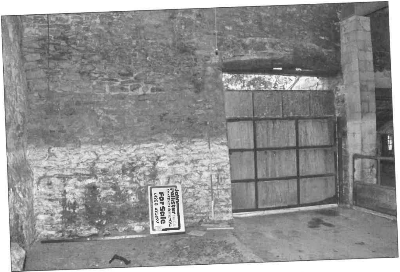
Photo 10: Interior of four-bay barn: west end, looking north-east
