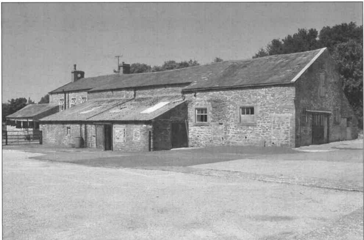
Photo 18: General view of barn range, from the south-east
