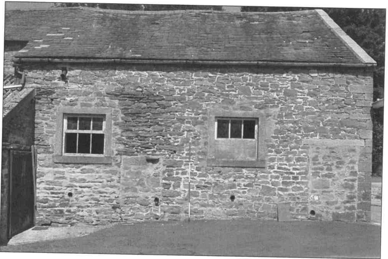
Photo 19: South side of east end of barn
