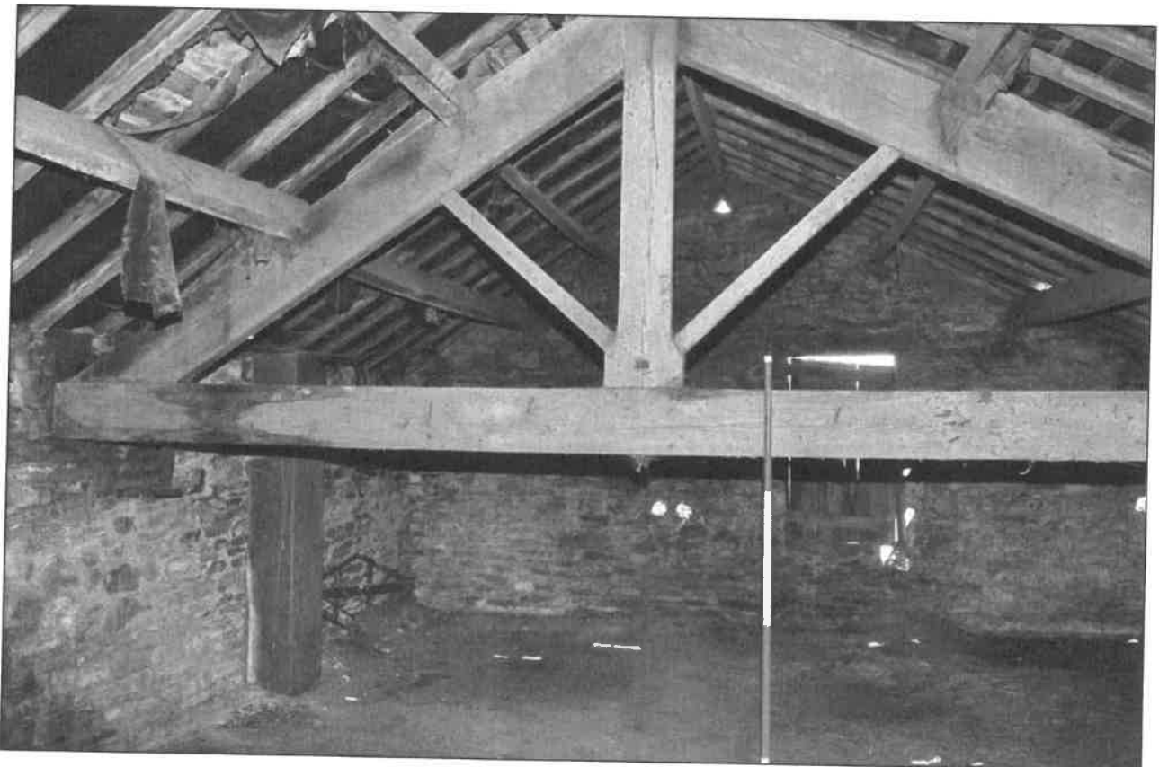
Photo 20: Hayloft and roof truss in east end of barn, looking east
