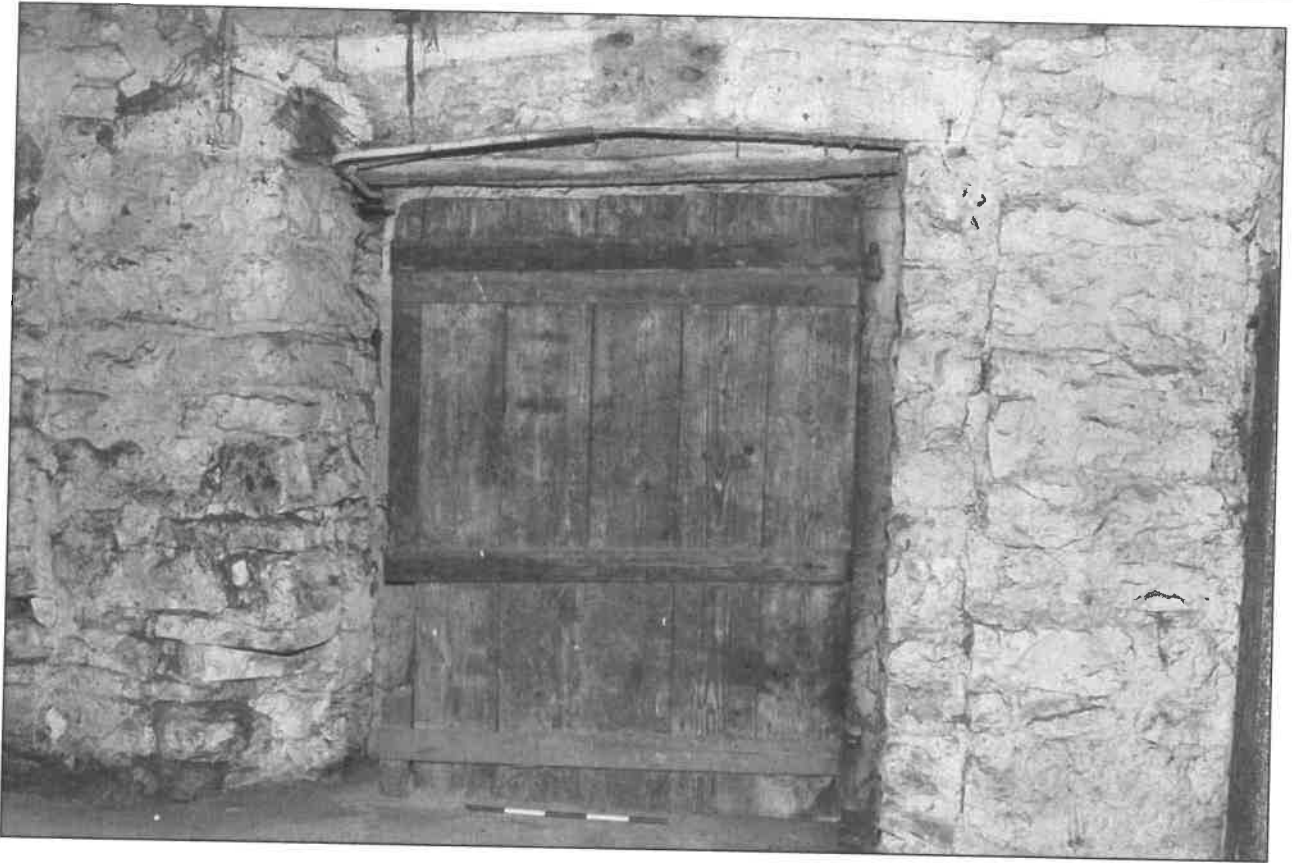
Photo 7: Inner face of winnowing doorway in south side of barn
