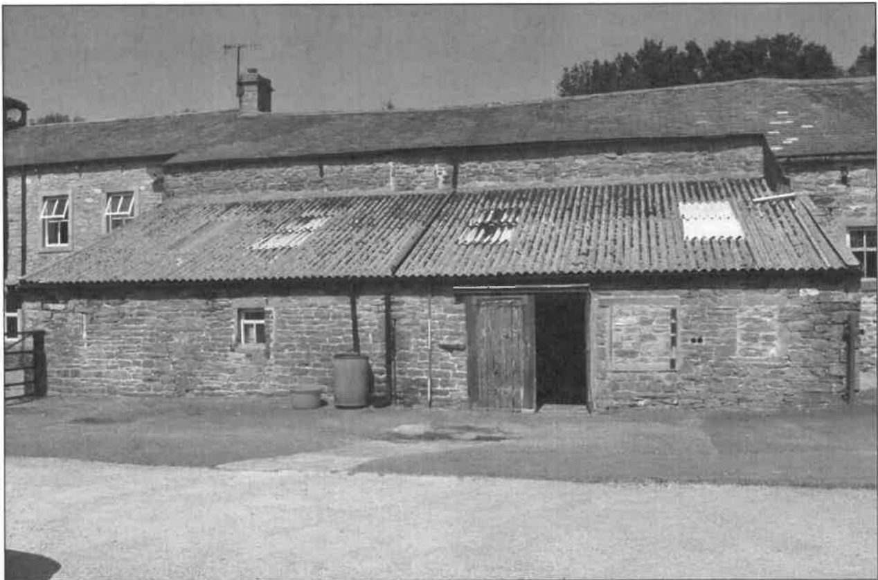
Photo 4: General view of the barn (west part) from the south
