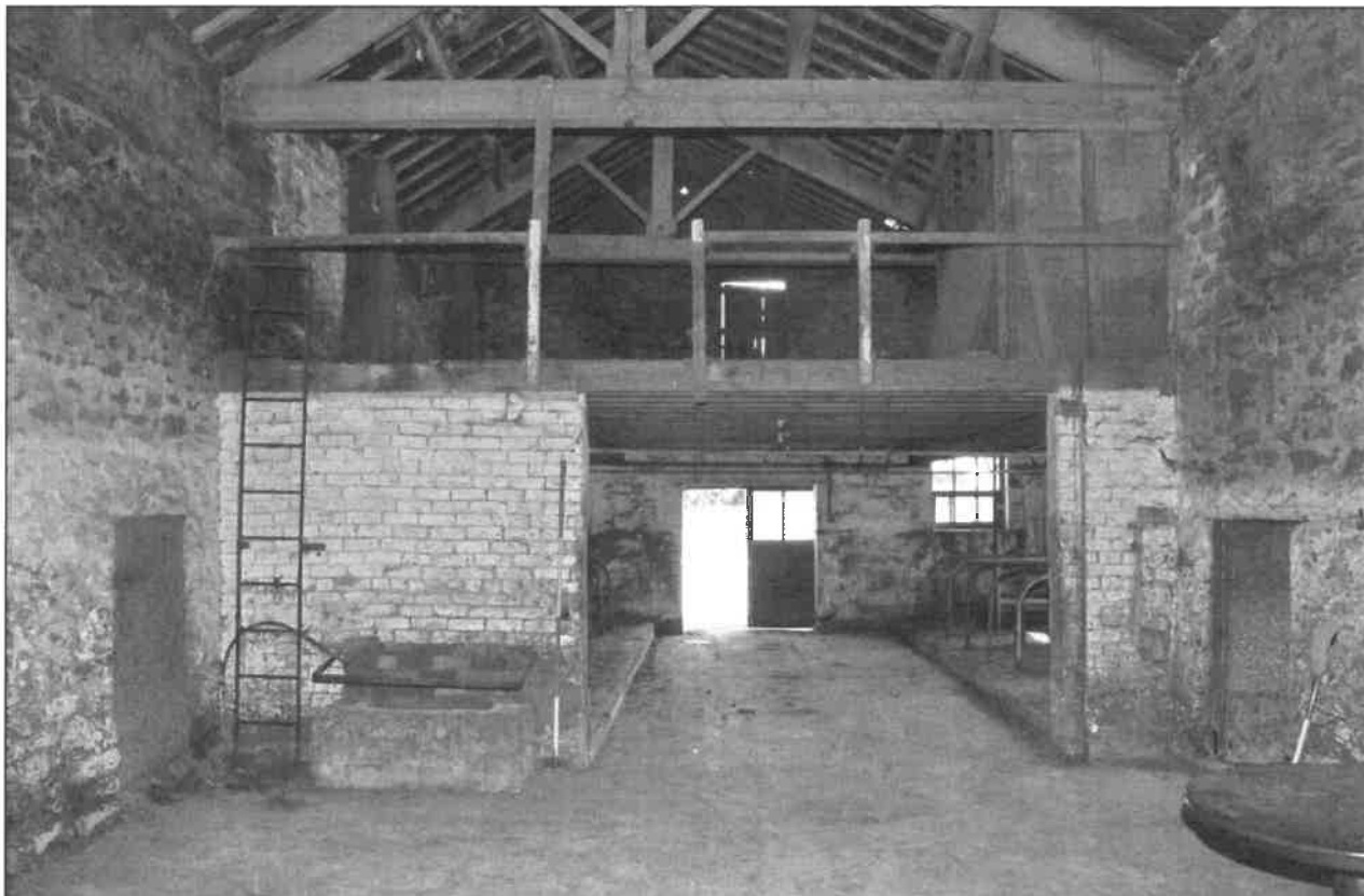
Photo 15: Interior of four-bay barn: east end, with extension beyond
