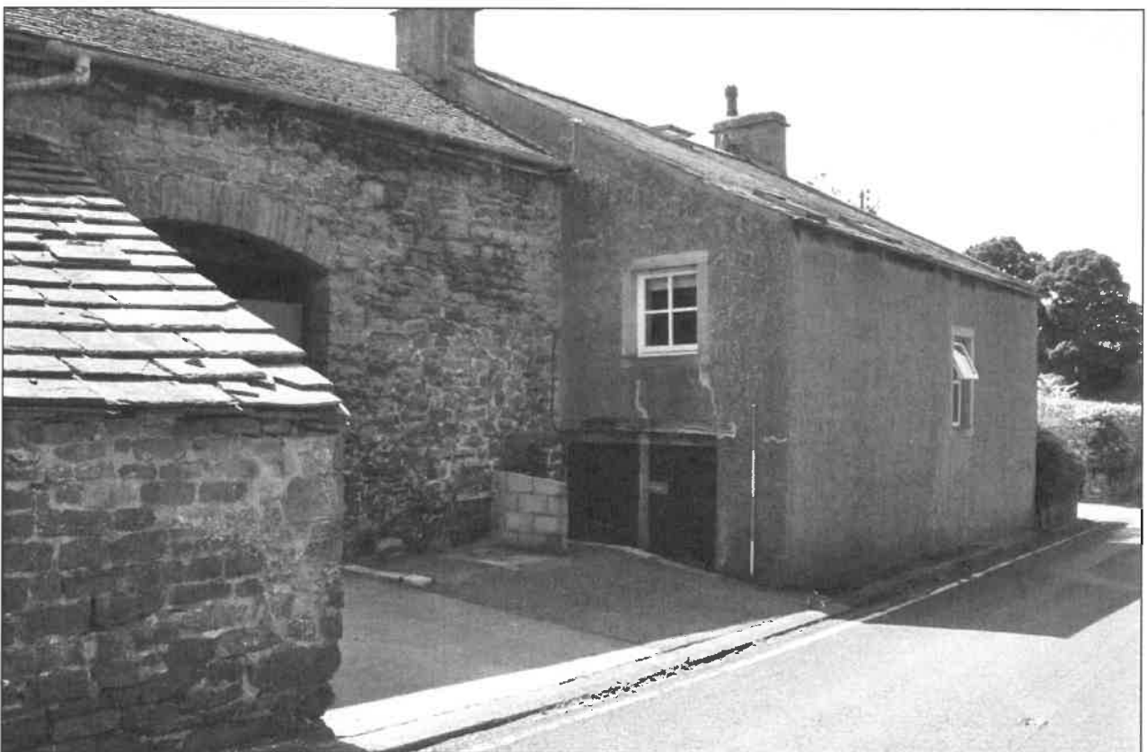
Photo 2: North side of barn, in relation to rear of farmhouse, looking south-west
