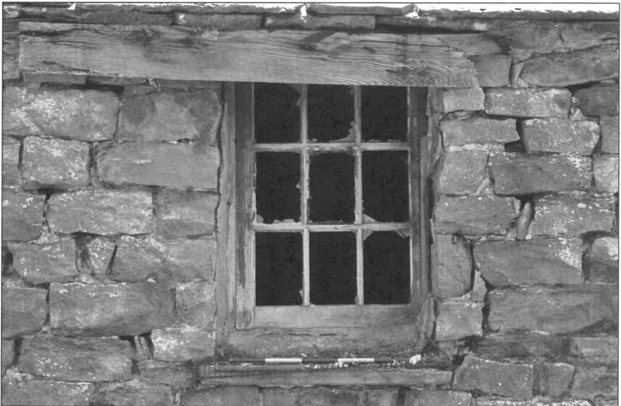
Photo 27: Detail of window in outshut on north side of barn
