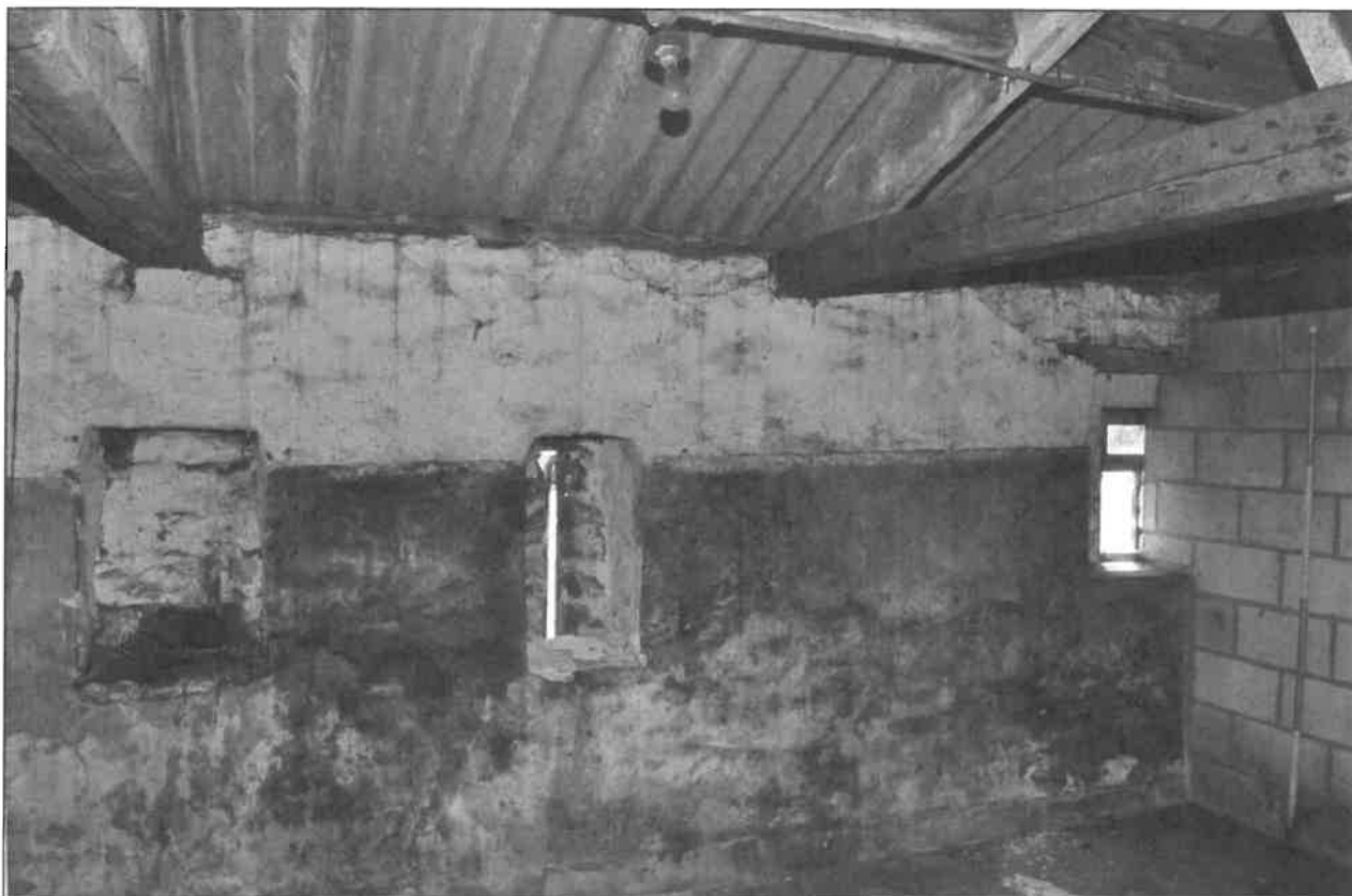
Photo 41: Outshut on south side of barn: interior, looking south
