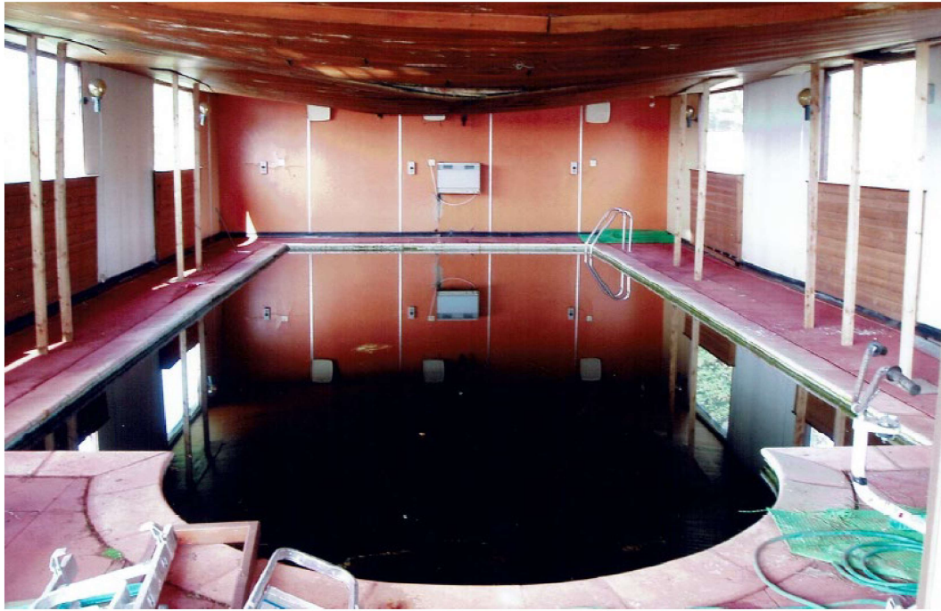
Fig 4. Evidence of Swimming Pool Roof Bowing Internally (Khan Family circa. 2006)
