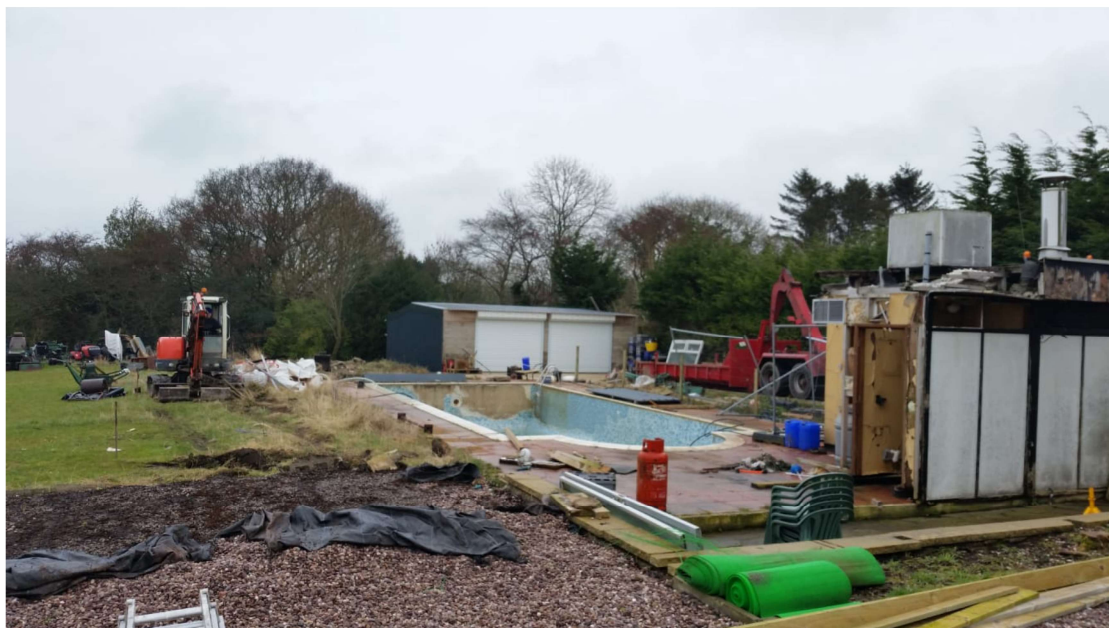
Fig 5. Removal of Collapsed Structure, Plant Room Remaining (Khan Family, March 2016)
