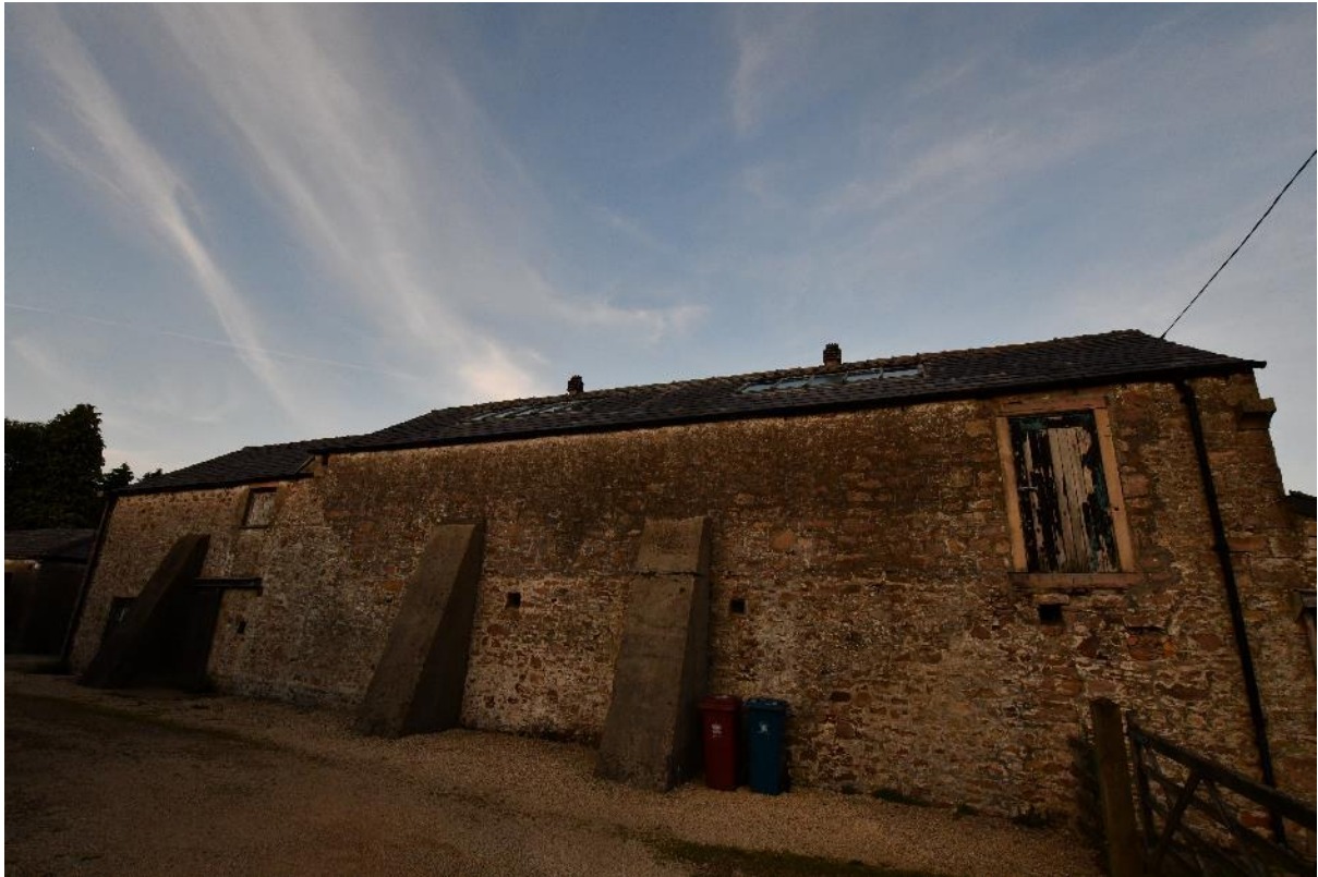
Image 5 Stone built barn with slate roof and skylights
