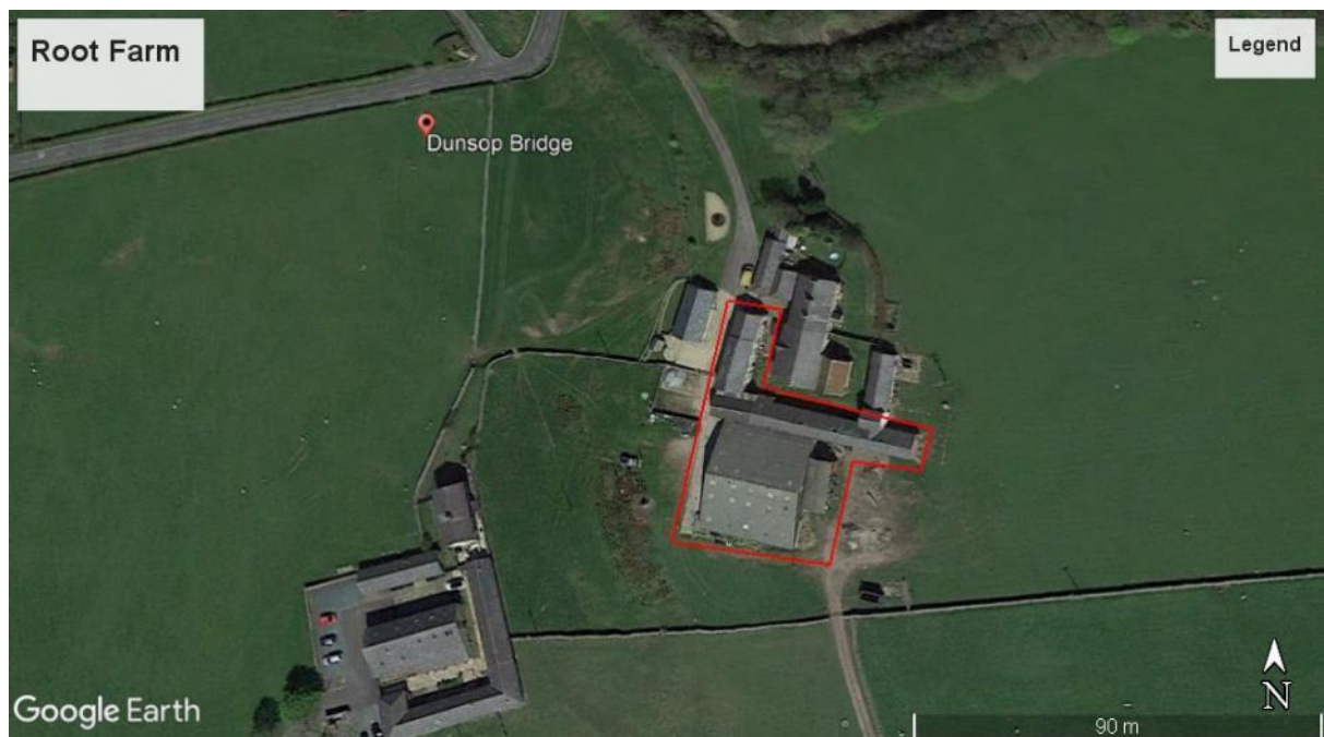
FIGURE 1. Site boundary indicated by the red line above.
