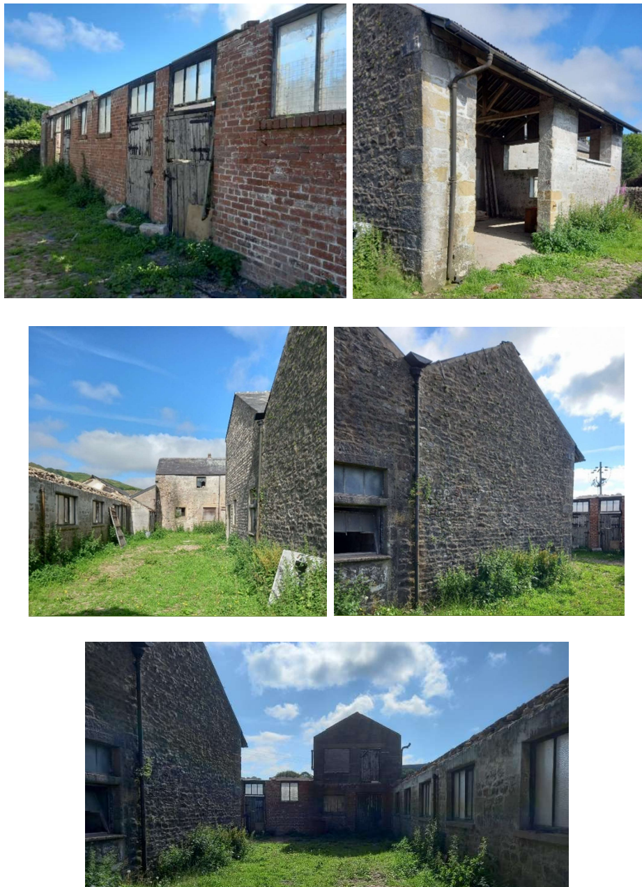
Fig. 10 Selected photos of the farm site (two storey buildings on middle row and in left hand side of bottom image not included in the application site)
