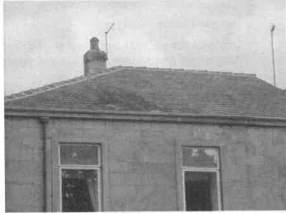
Photo 4: Slate covered roof above Flat 8 (southern elevation)
