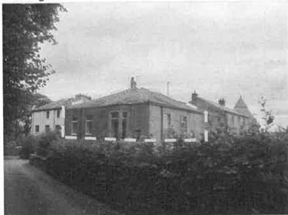
Photo 3: Western and southern elevations and slated covered hipped roof
