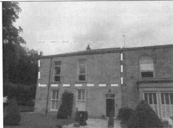
Photo 1: Southern elevation of section of building showing Flat 8
