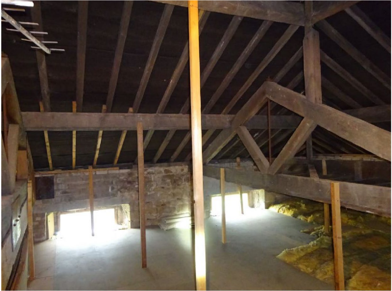
fig 2. Internal view of windows W01 and W02 and shown on elevational drawing.
