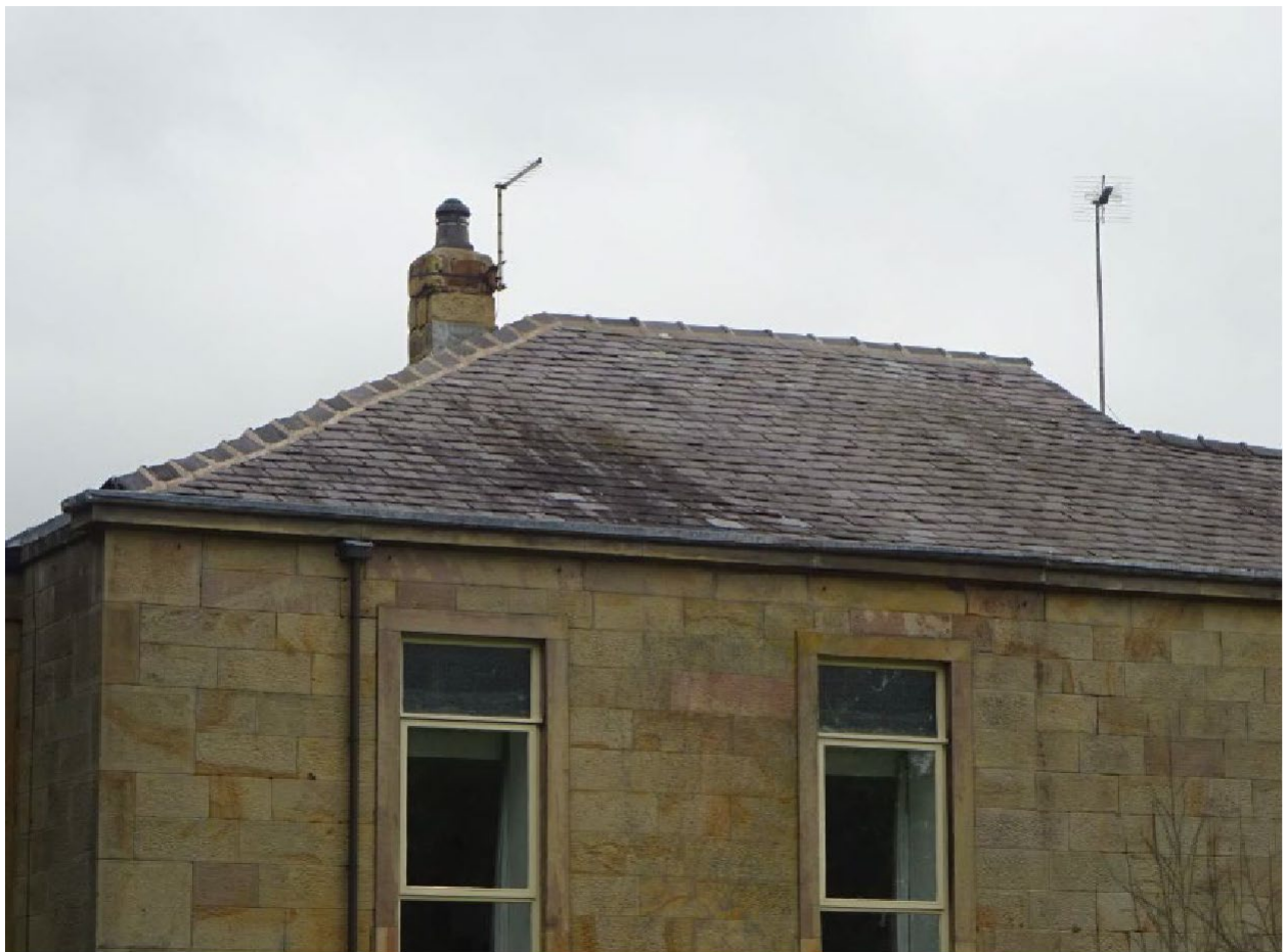
fig 2. Photograph showing the existing flat ceiling visible externally through the existing windows.
