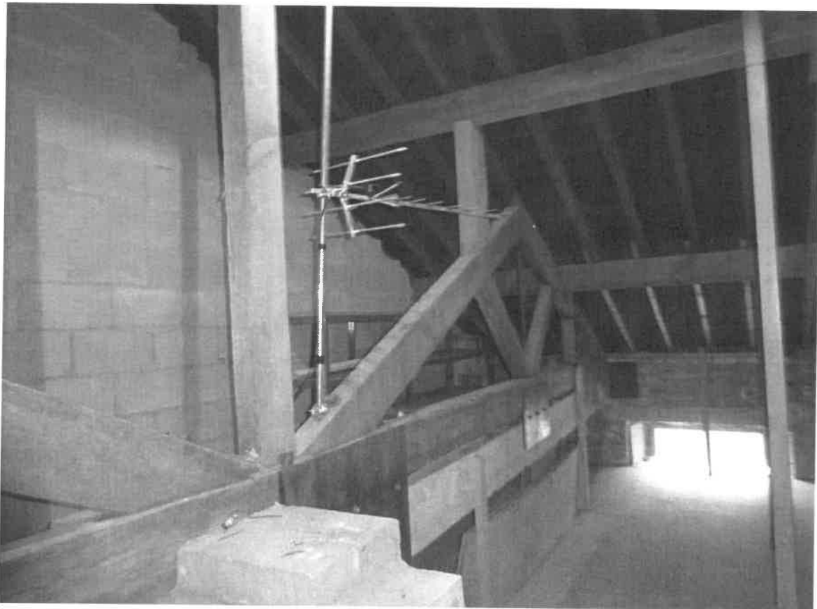
Roof Void – Original roof trusses / steel plates / ceiling hangers
