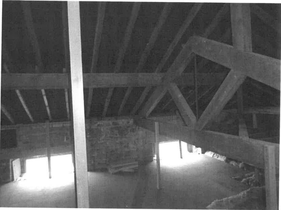
Roof Void – Original roof trusses / steel plates / ceiling hangers
