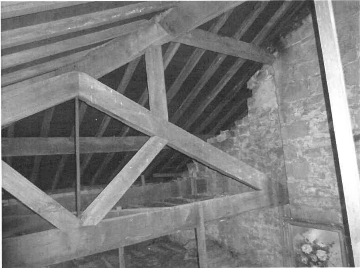
Roof Void – Original roof trusses / ceiling hangers
