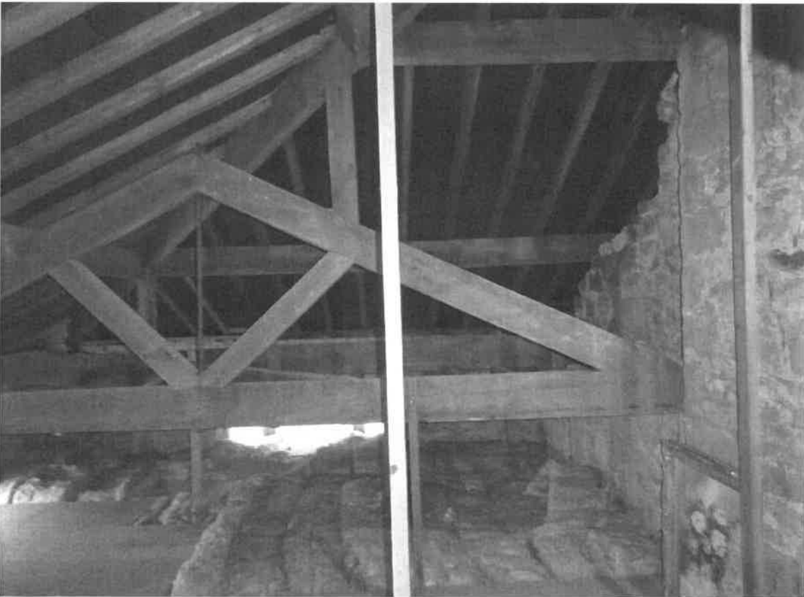
Roof Void – Original roof trusses / ceiling hangers
