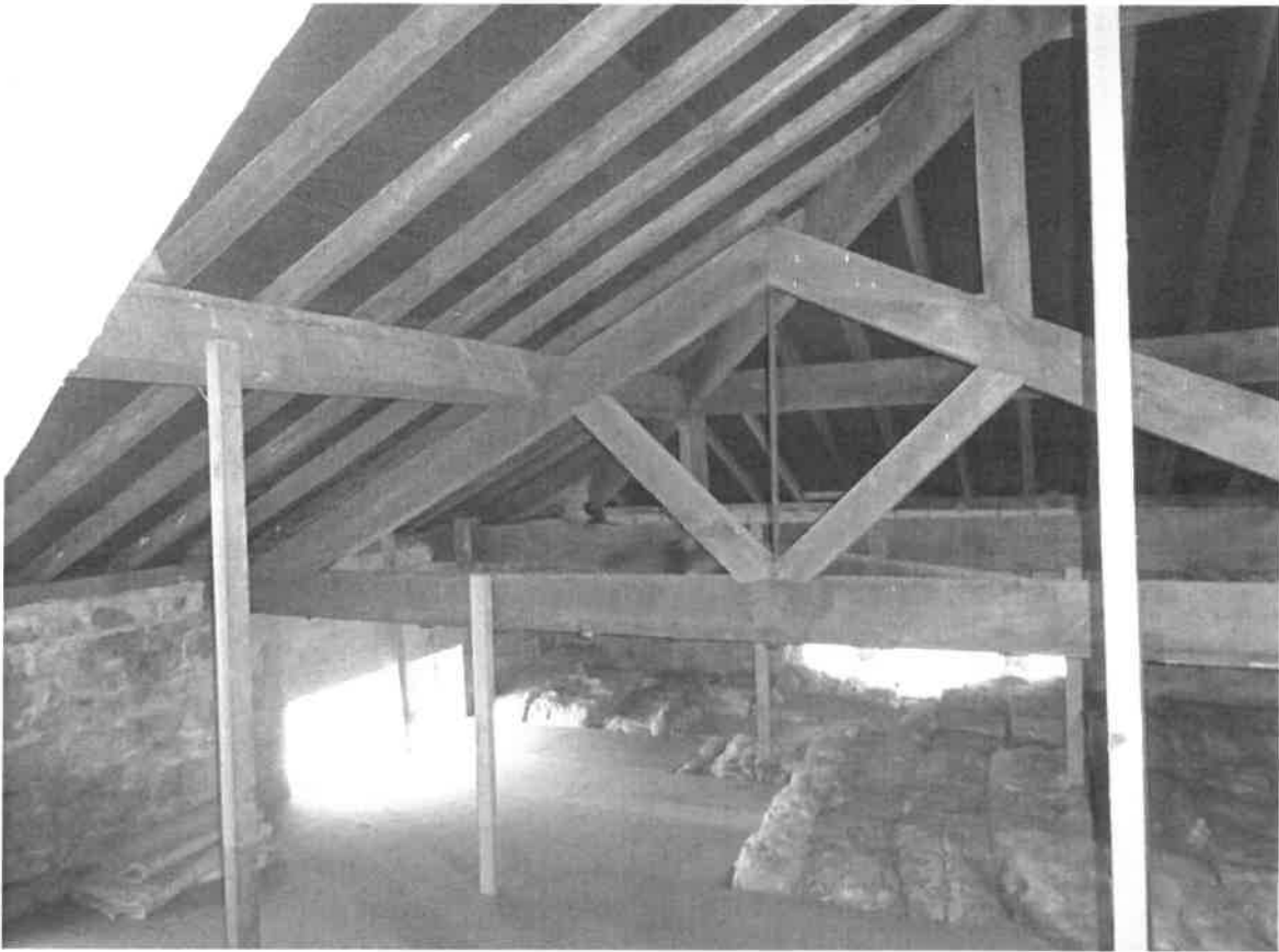
Roof Void – Original roof trusses / ceiling hangers
