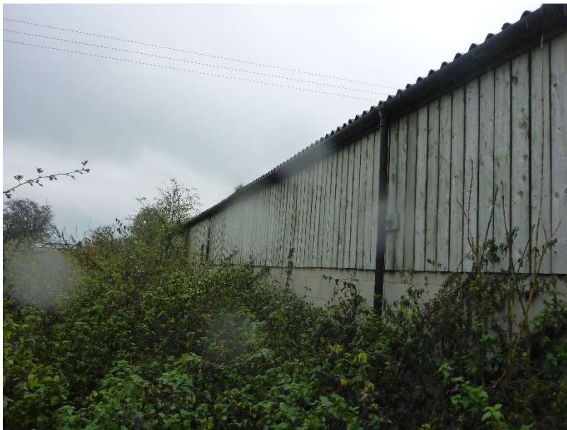
Photo 4: Eastern Elevation of the Agricultural Building showing Largely overgrown vegetation.
