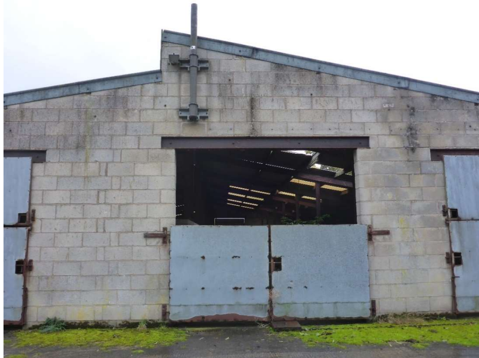
Photo 2: North Elevation of the Agricultural Building showing split level roof
