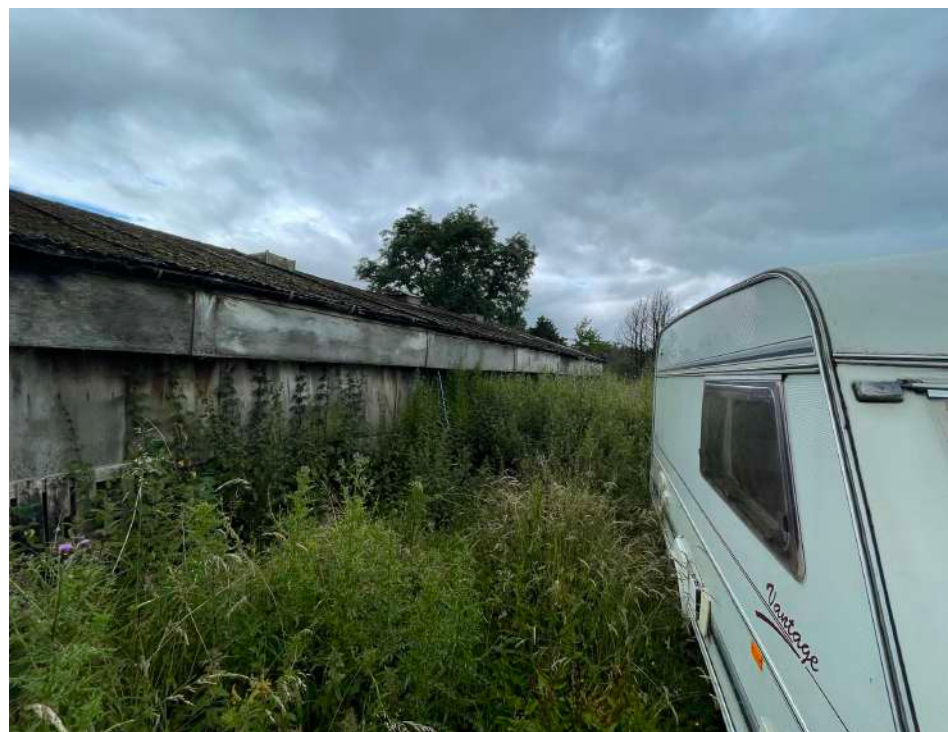
Side view of existing storage building
