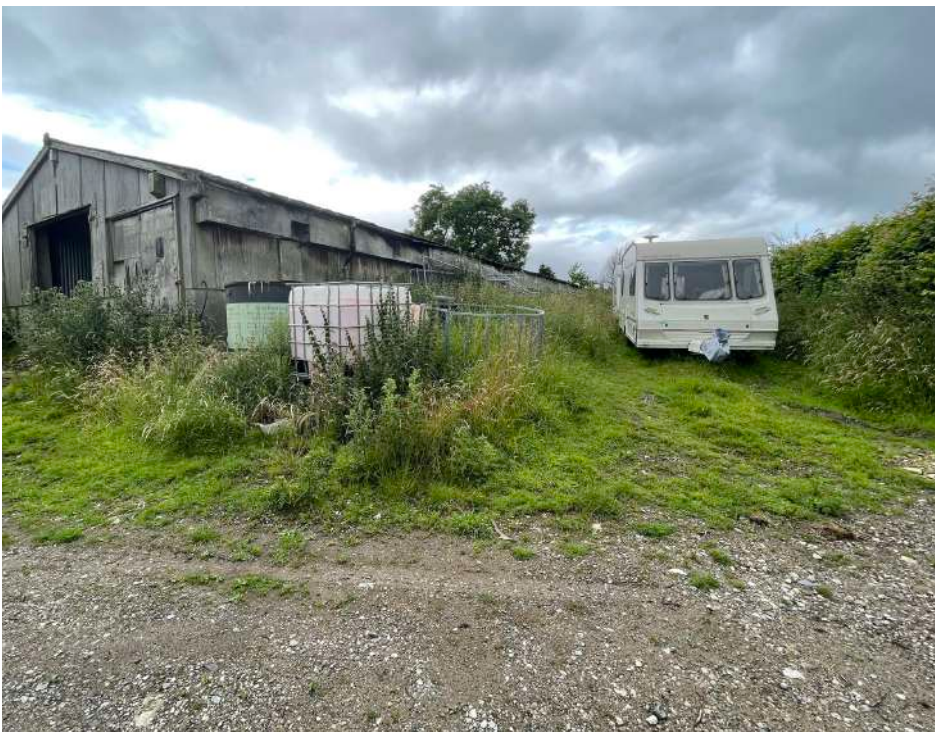
Side view of existing storage building
