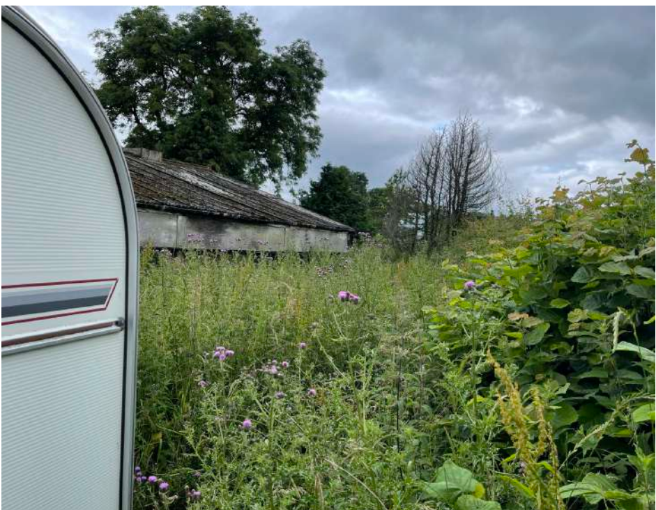
Side view of existing storage building
