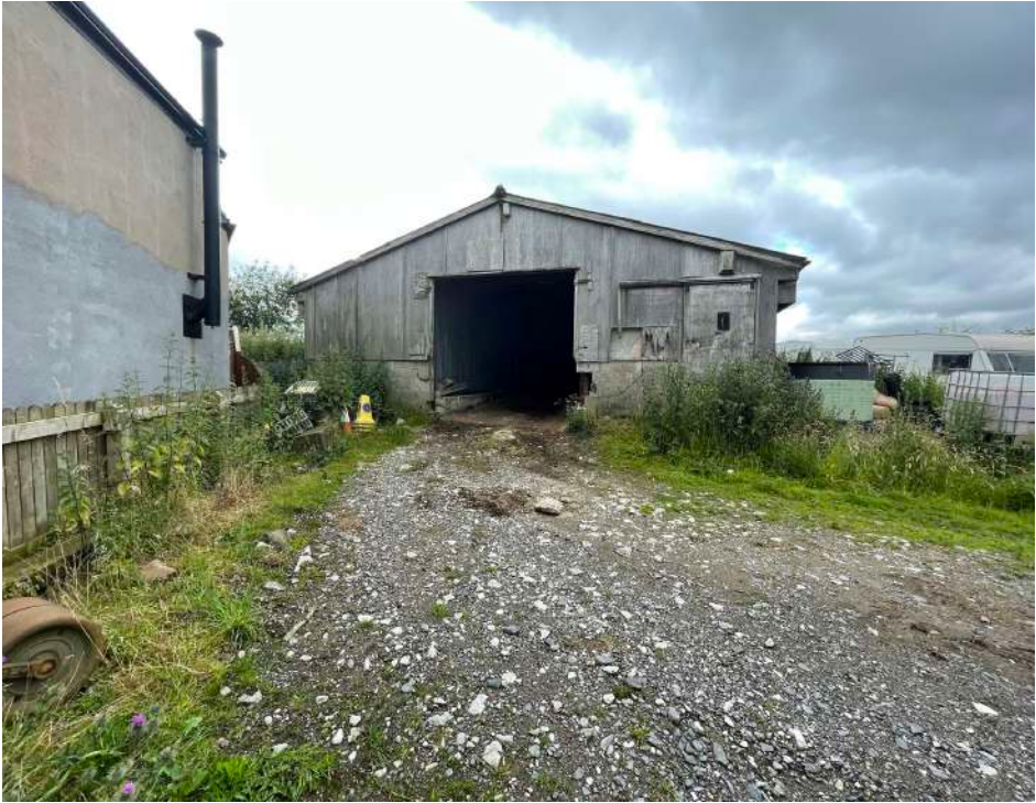
Front elevation of existing storage building
