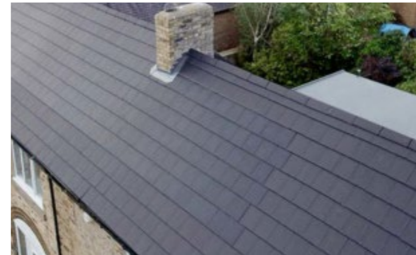
Slate Grey Solecco Solar PV Tiles (As Proposed for the SE Roof of Courtyard Building)
