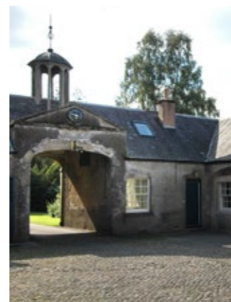
Stables Cottage Hendersyde
