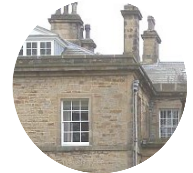
Parapet and cornice at Downham Hall
