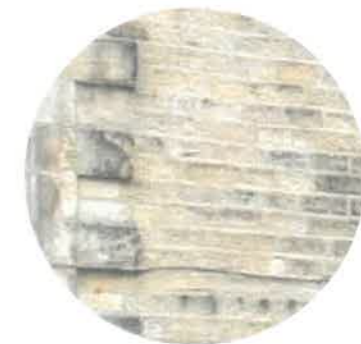
Reference to the projecting quoins at Whins Hall, Sabden (Grade II Listed)
