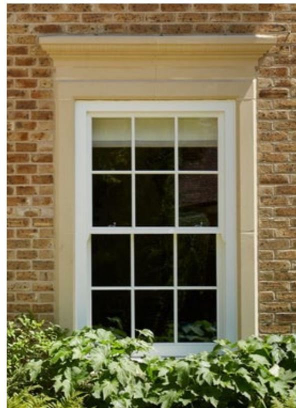
Painted timber sash window
