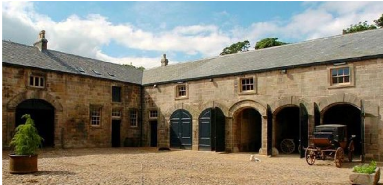
Gibside Stables, Newcastle
