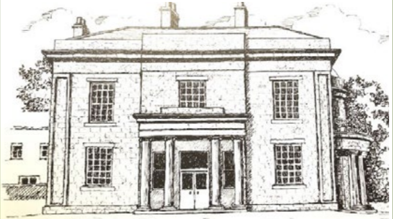
Read Hall's simple tall parapet with large projecting cornice. Central projecting bay and portico
