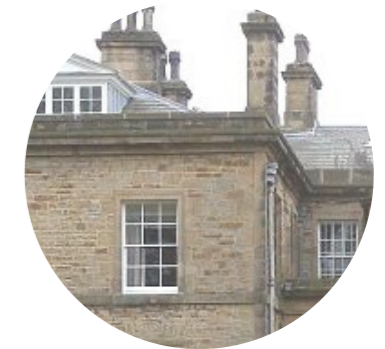
Parapet and cornice at Downham Hall
