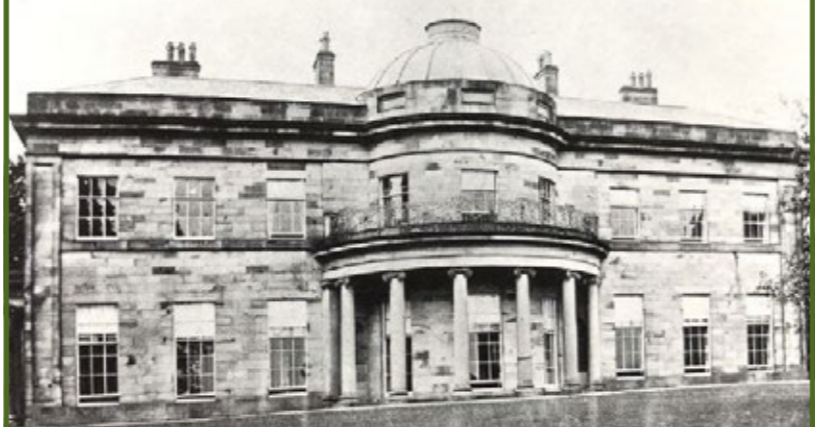
Read Hall's bowed portico with Ionic order colonnade and balcony above. Tall, plain solid stone parapet
