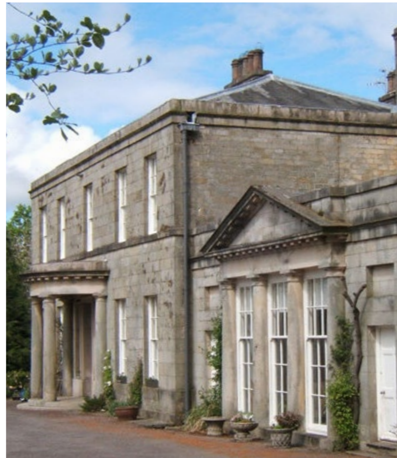
Bowed Portico & Orangery at Casterton Hall, Kirkby Lonsdale (Grade II Listed)
