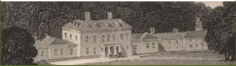
Read Hall's simple tall parapet with large projecting cornice. Central projecting bay and portico
