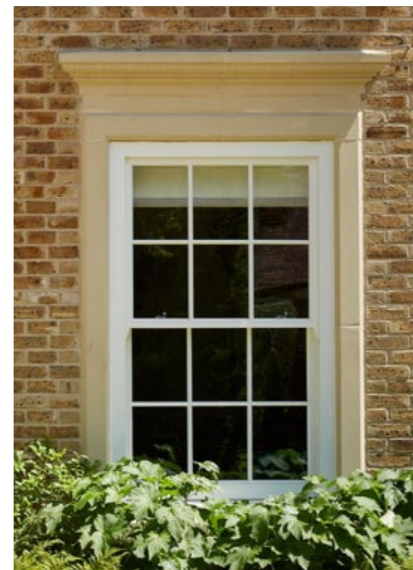
Painted timber sash window
