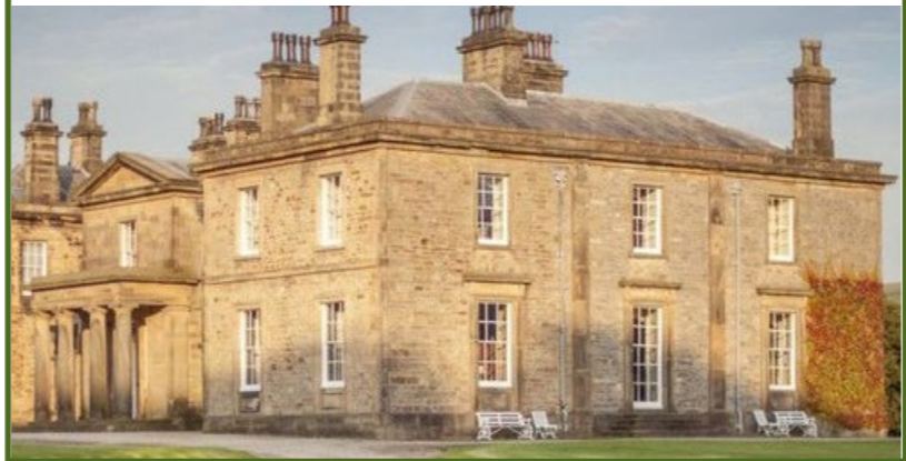
Broughton Hall showing George Webster's iconic 'Porte Cochere'. To the left, a simple unadorned pediment over recessed ionic order central feature
