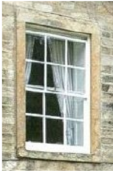
Stone heads and jambs with sliding sash window, Whins House, Sabden
