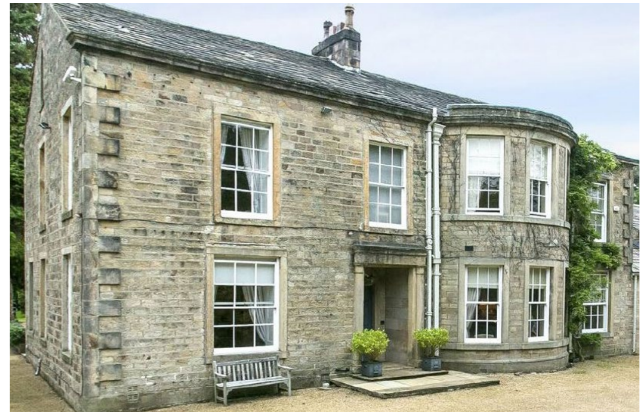
Whins House, Sabden (Grade II Listed)
