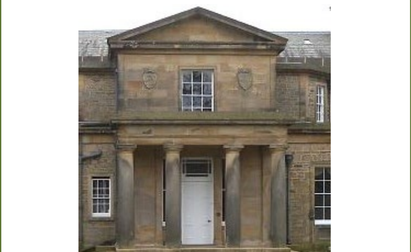
Downham Hall's plain Roman pediment, no decoration above central window and 4 Greek Doric columns
