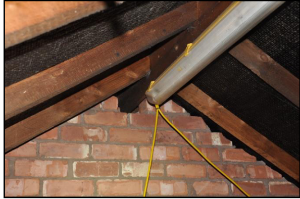
Internal view of roof void, plaster board section (lhs) and underlined section (rhs) showing connecting gaps at wall top between adjoining properties
