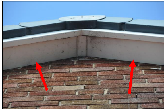
View of tight-fitting roof coverings (lhs) and view of gaps associated with soffit at the gable, indicated by red arrows (rhs)
