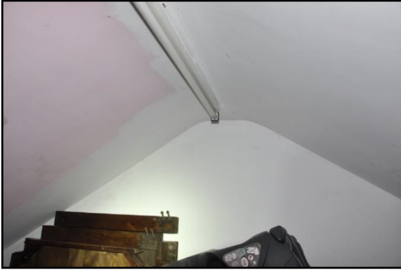
Internal view of roof void, plaster board section (lhs) and underlined section (rhs) showing connecting gaps at wall top between adjoining properties
