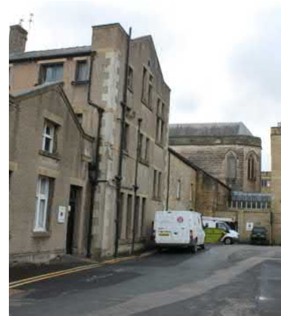
View of north elevation and service road
