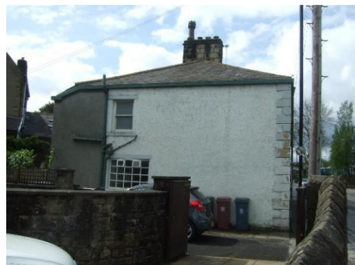
Picture 5 - North elevation
