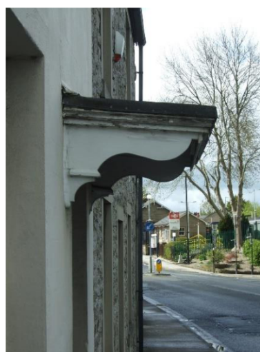
Picture 9 - Timber hood to #13
