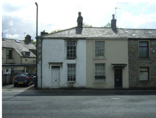
Picture 4 – West elevation along Railway View Road
