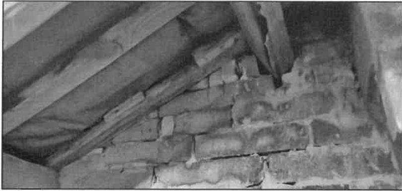
Photograph 8 showing cavities in the brickwork around the timber
