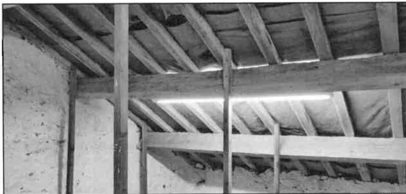
Photograph 7 showing the roof joists
