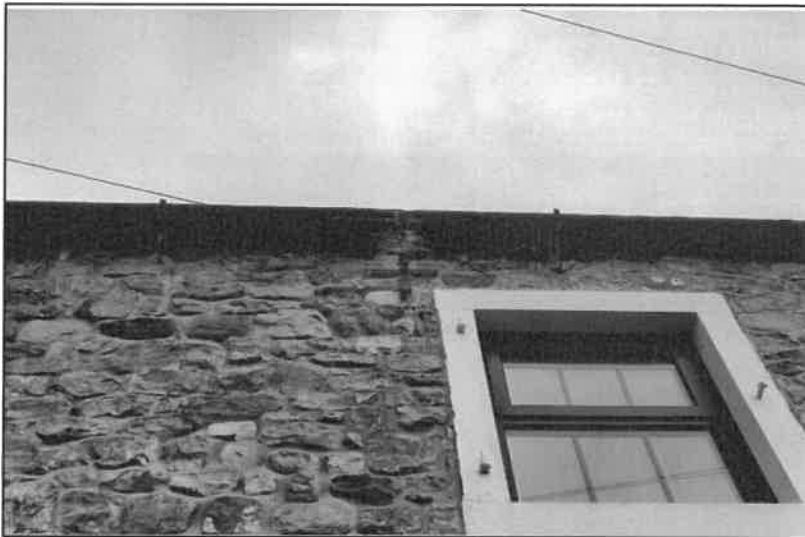
Photograph 4 showing a gap underneath the eaves of the roof
