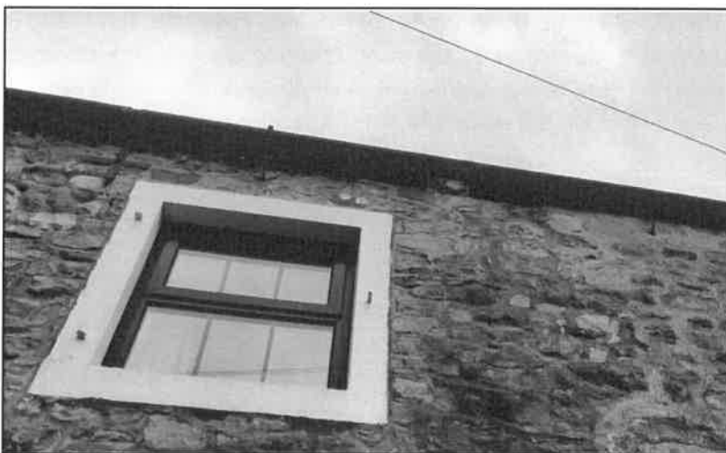
Photograph 5 showing another gap underneath the eaves of the roof
