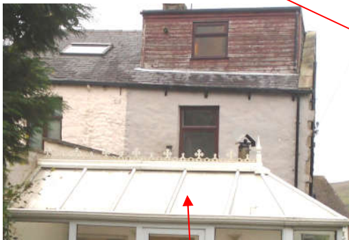
The Conservatory roof is clear polycarbonate sheets and upvc frame.
