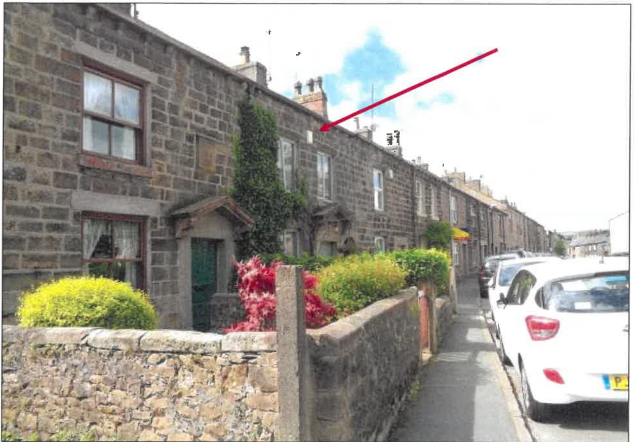
1. The application property within its terrace, looking north along Church Street
