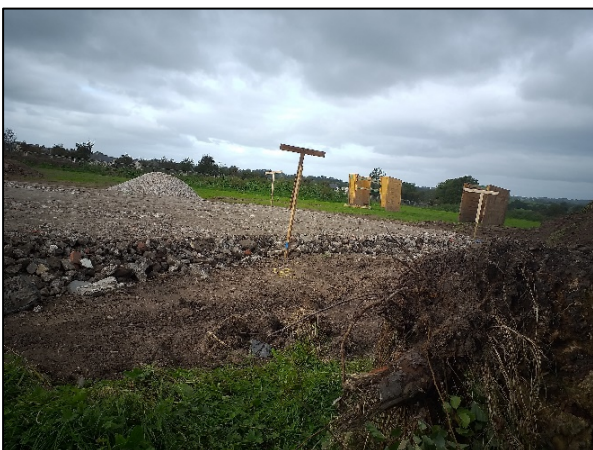
Photograph 3 – Construction activity within site
