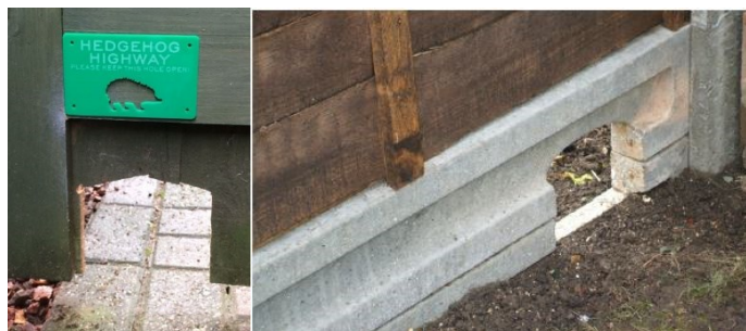
Insert 3: Showing wildlife access gap within fencing
