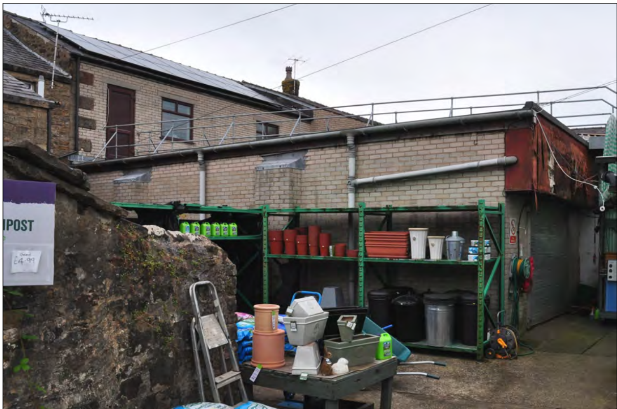
Photo 4: Rear of front block, with modern single storey rear wing
