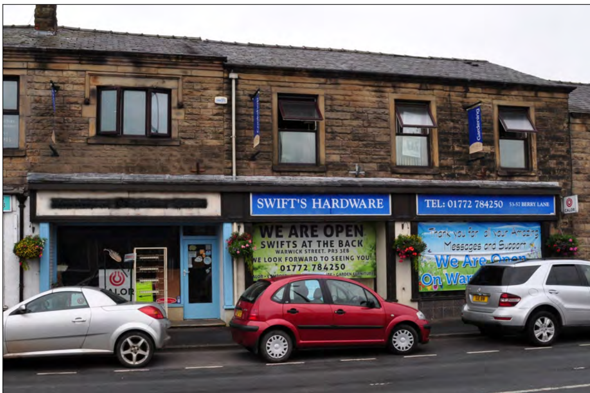
Photo 2: Berry Lane frontage
