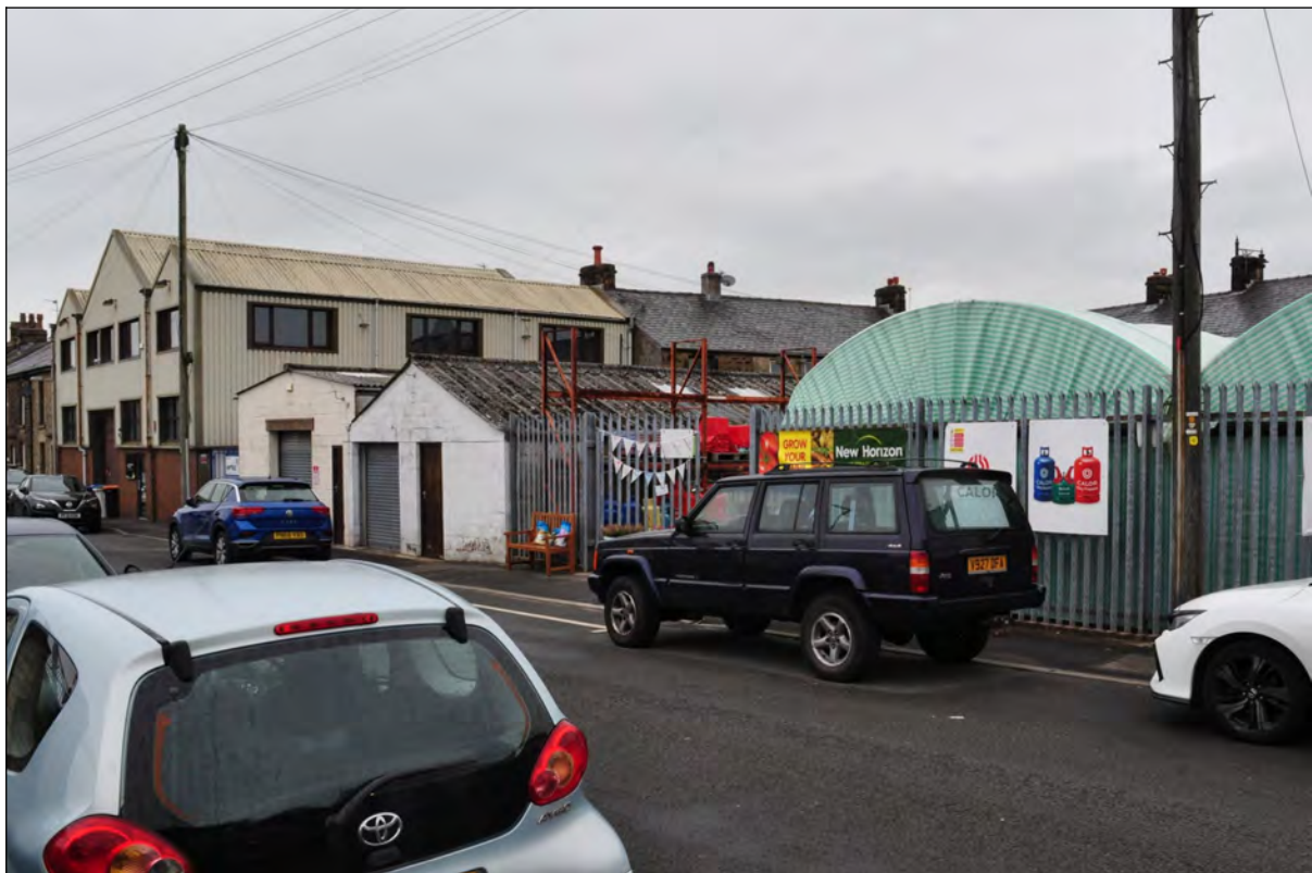
Photo 6: South-west part of site, along Warwick Street
