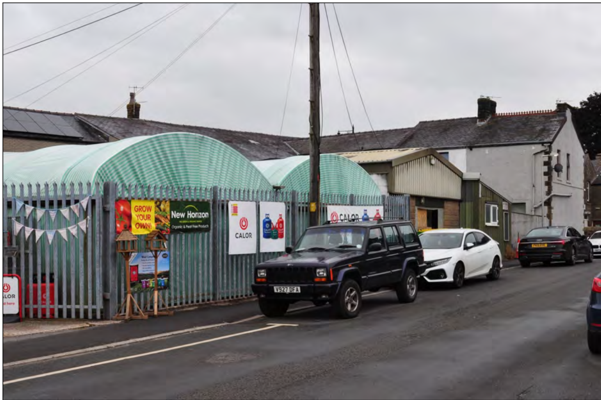
Photo 5: South-east part of site, along Warwick Street
