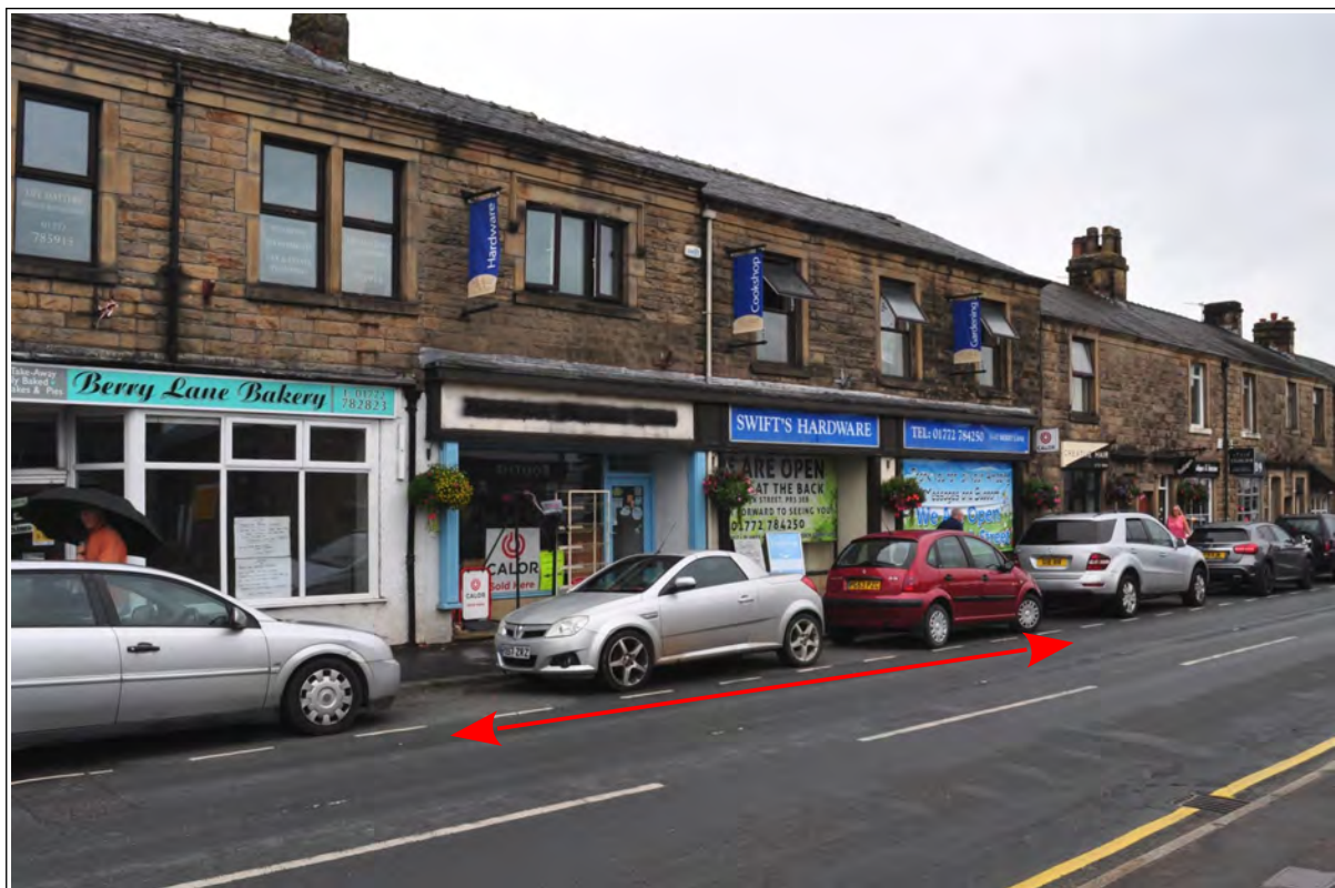
Photo 1: Berry Lane frontage
