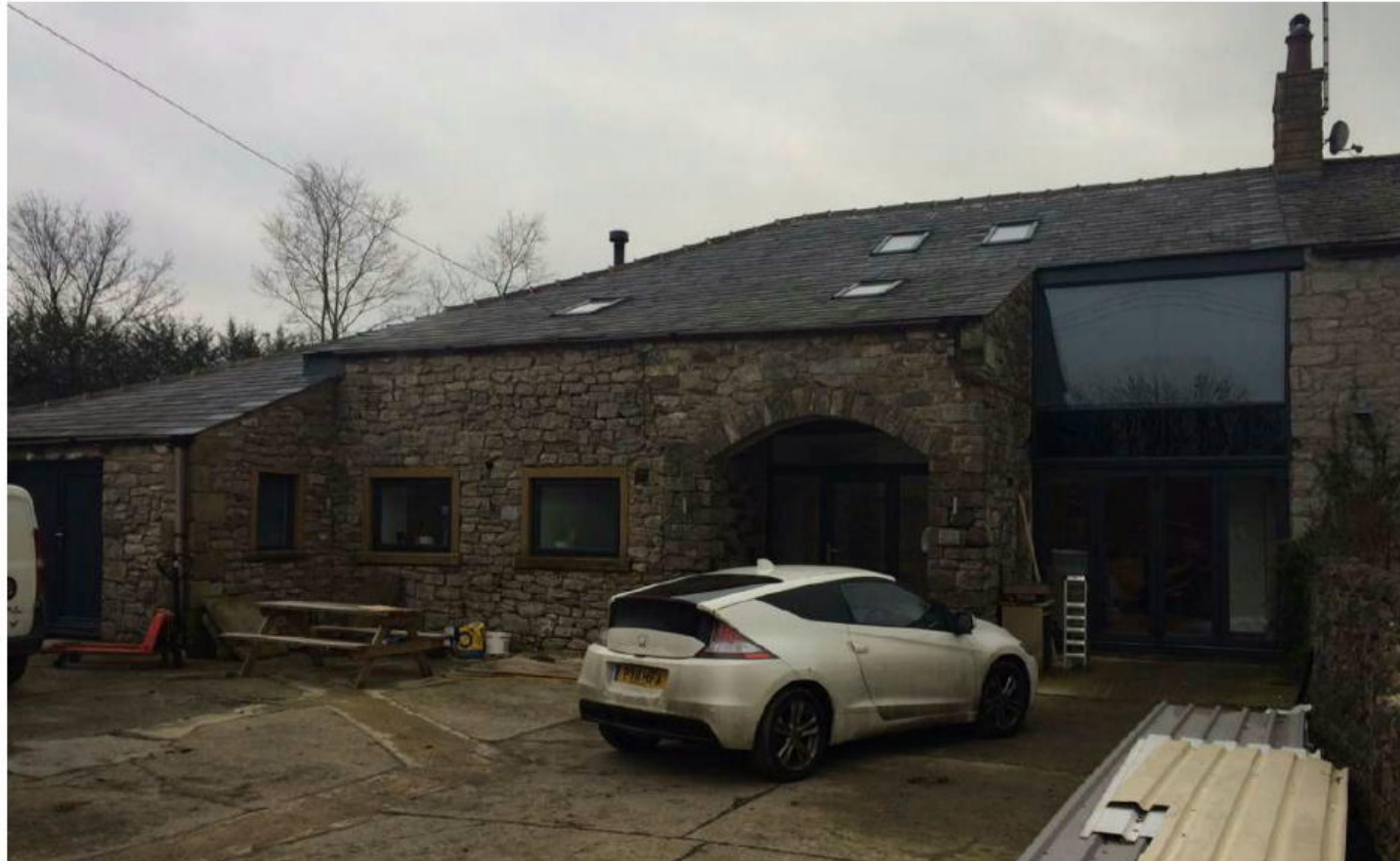
PL02: Photograph of Twinbrook Barn (west elevation)
