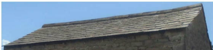
photograph (1) - North pitch of 2 storey stone outbuilding
