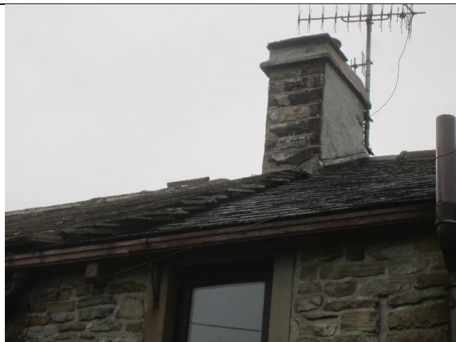
Photo 8: Join between stone tile roof covering at the off-site building and Pentangle Barn
