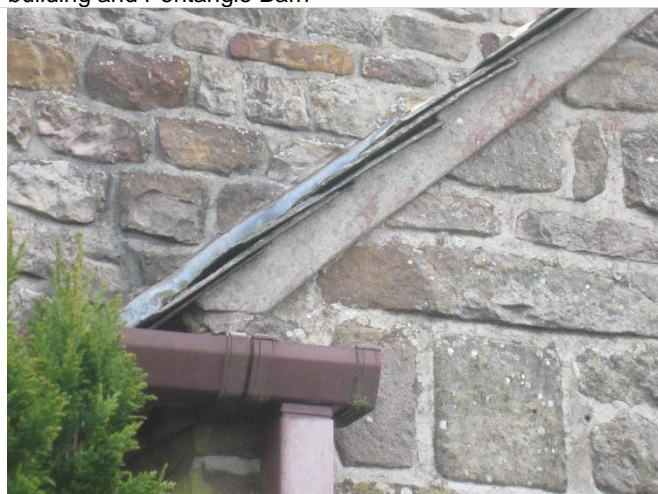
Photo 10: Gaps at the roof verge on the porch attached to the northern (front) elevation of Pentangle Barn (Building 1)
