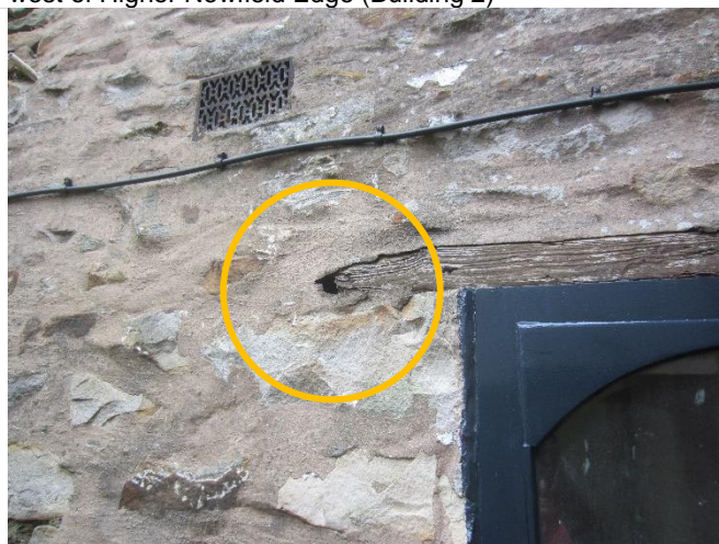
Photo 16: Gap in the stonework at the eastern elevation of Higher Newfield Edge (Building 2). Inspection with an endoscope confirmed only extends 0.08 metres into the wall; no bats or bat droppings found.
