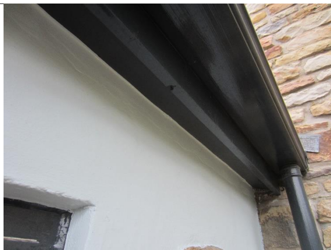
Photo 14: Sealed soffits at single storey side extension to the west of Higher Newfield Edge (Building 2)
