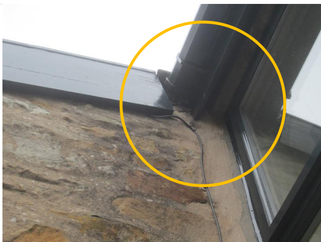
Photo 17: Gap behind fascia at eastern elevation of Higher Newfield Edge (Building 2). Inspection with an endoscope carried out; no bats or bat droppings found.
