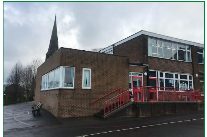
The southwest and northwest elevation of the school – showing the single-storey extension that will be extended upwards.
