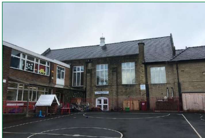
The northwest elevation of the school – showing how the two-storey flat-roofed extension attaches to the main body of the school
