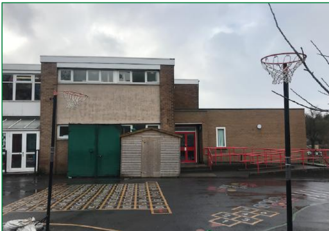
The northeast elevation of the school – showing the two-storey and single-storey flat-roofed extension
