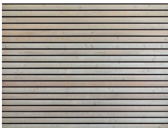
HORIZONTAL LARCH CLADDING
