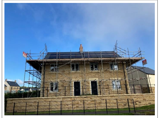
Source: CBRE Ltd.
