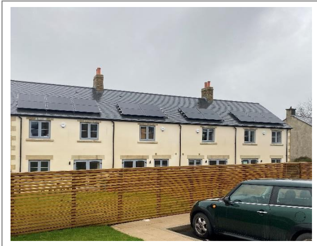
Source: CBRE Ltd.
