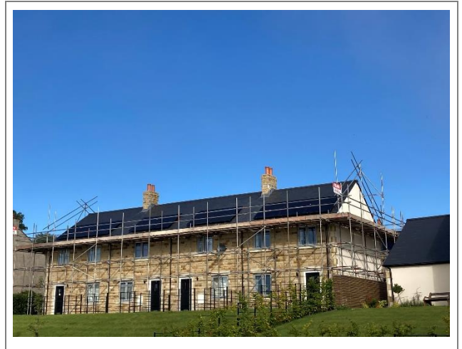
Source: CBRE Ltd.
