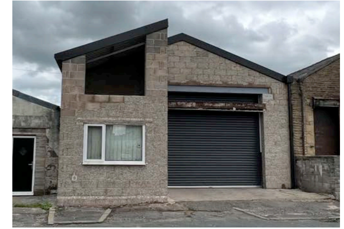
current 'as built' photograph - work ceased
