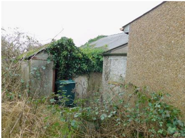
PHOTO 17 North-western Corner of Bungalow
