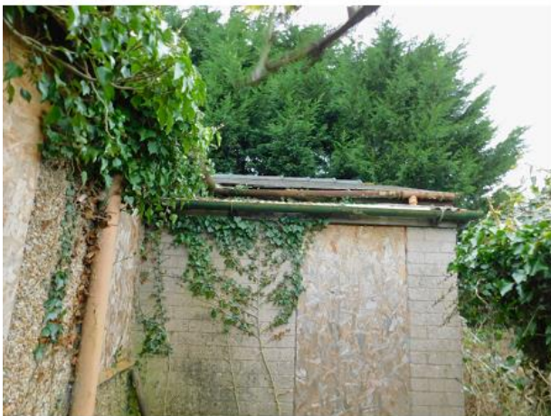
PHOTO 21 Eastern Elevation of Utility Extension
