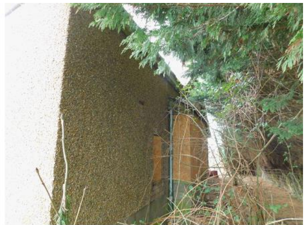
PHOTO 14 North-western Corner of Kitchen Elevation
