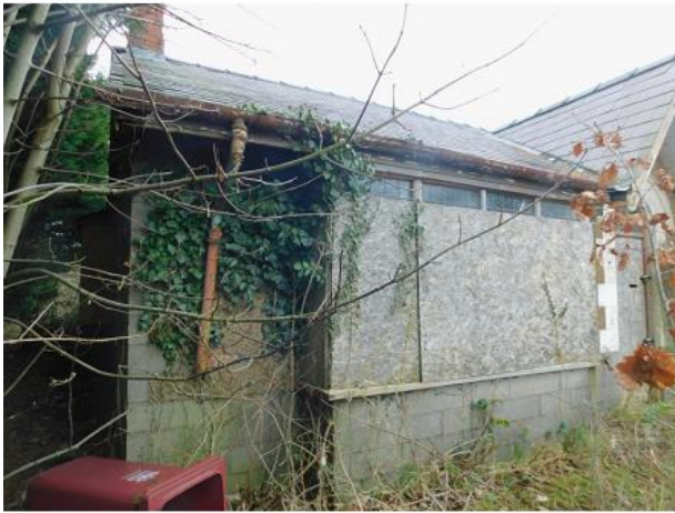
PHOTO 9 South-western Corner of Bungalow
