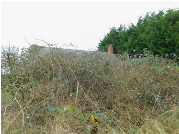
PHOTO 23 Northern Elevation of Bungalow
