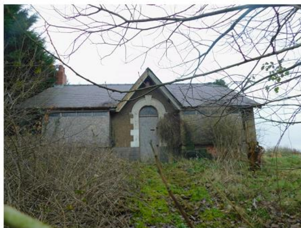
PHOTO 6 Southern Elevation of Bungalow
