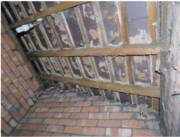
PHOTO 25 Underside of Extension Roof
