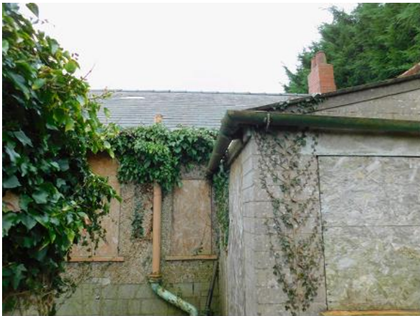
PHOTO 19 Part Northern Elevation of Bungalow
