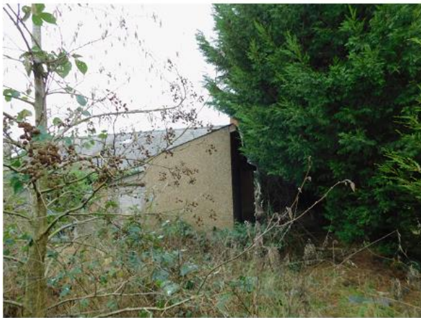
PHOTO 15 Northern Elevation of Kitchen Extension
