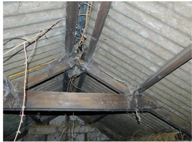
PHOTO 32 Underside of Outbuilding Roof
