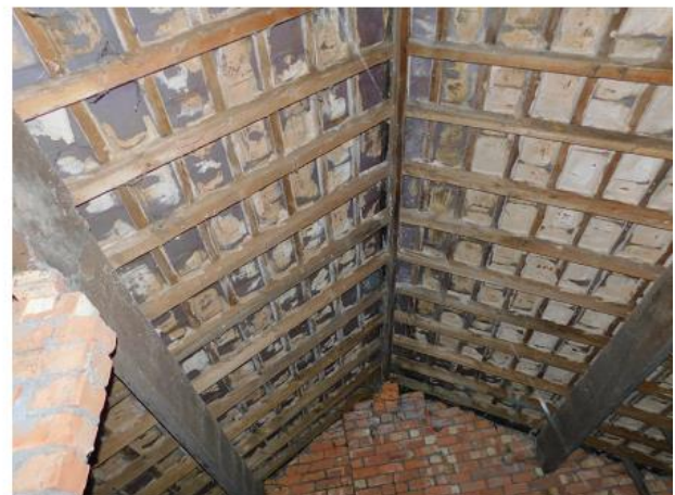
PHOTO 24 Underside of Bungalow Main Roof
