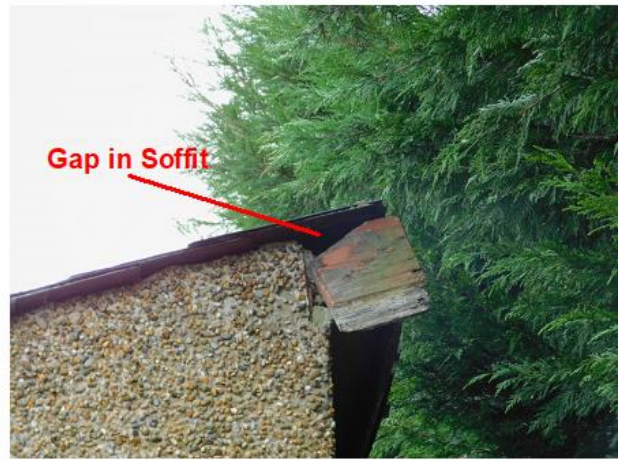
PHOTO 16 North-western Corner of Kitchen Extension
