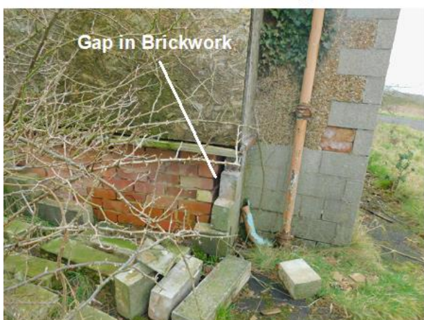
PHOTO 3 Part South-eastern Corner of Bungalow
