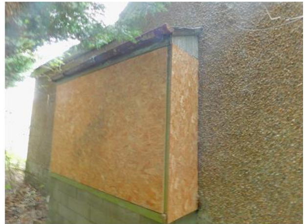
PHOTO 12 Western Elevation of Kitchen Extension
