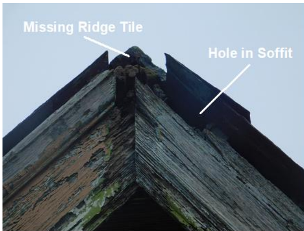
PHOTO 7 View of Entrance Roof
