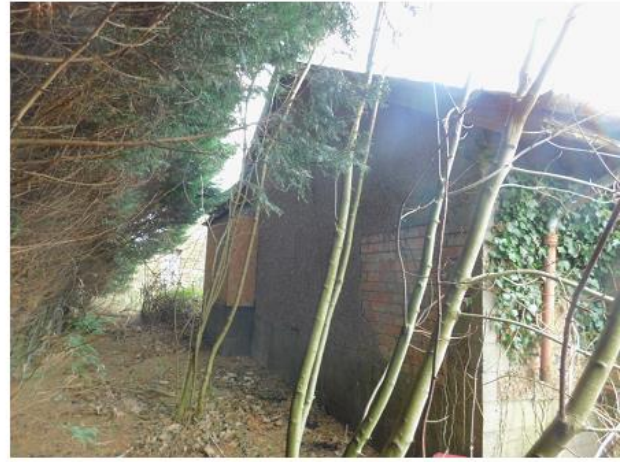
PHOTO 10 View Along Western Elevation
