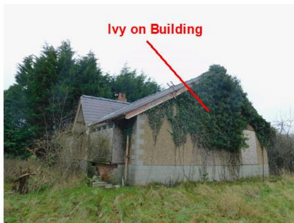
PHOTO 2 South-eastern Corner of Bungalow
