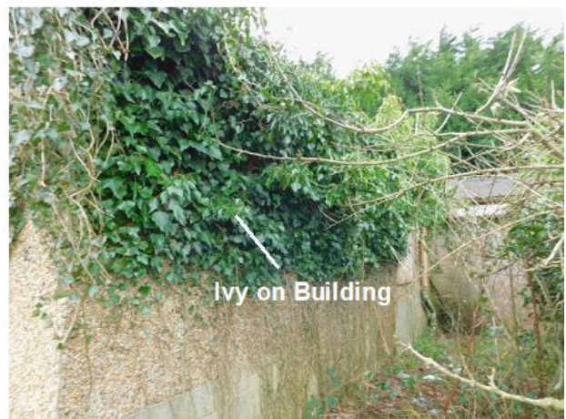
PHOTO 22 View Along Northern Elevation of Bungalow
