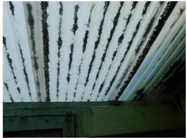
PHOTO 26 Underside of Utility Building Roof
