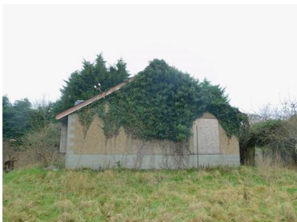
PHOTO 1 Eastern Elevation of Bungalow
