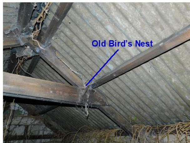
PHOTO 33 Southern Part of Outbuilding Roof
