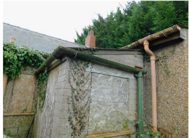
PHOTO 18 North-eastern Corner of Utility Extension
