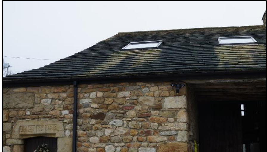
Photo 2: Roof area of barn on the southeast pitch.
