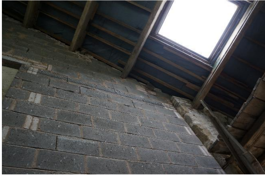
Photo 4: Internal view of roof structure and adjoining interior wall.
