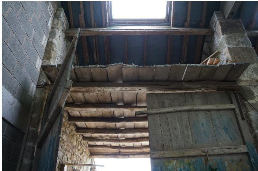
Photo 5: Internal view of the entrance porch viewed from inside the barn.
