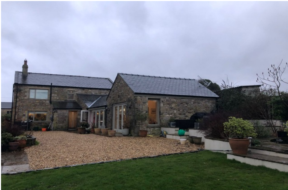
View of the application site and previous extension/alteration work
