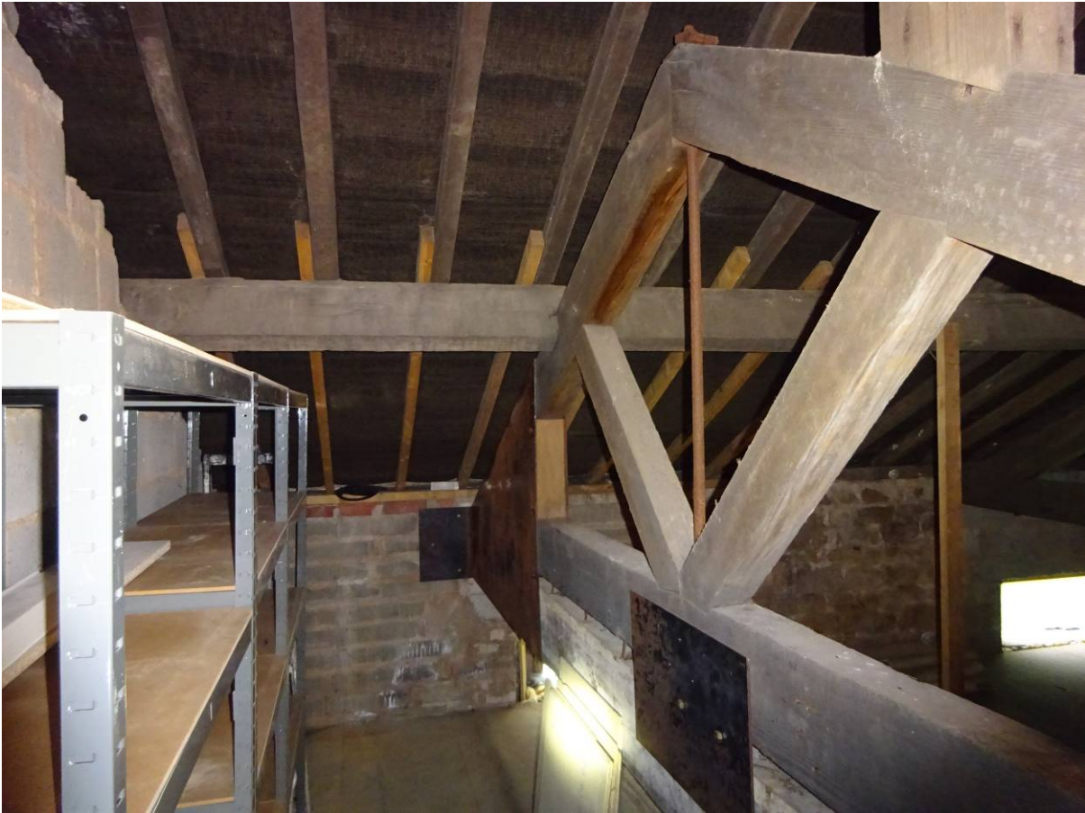
Roof Void – Original roof trusses / steel plates / original & replaced rafters / ceiling hangers
