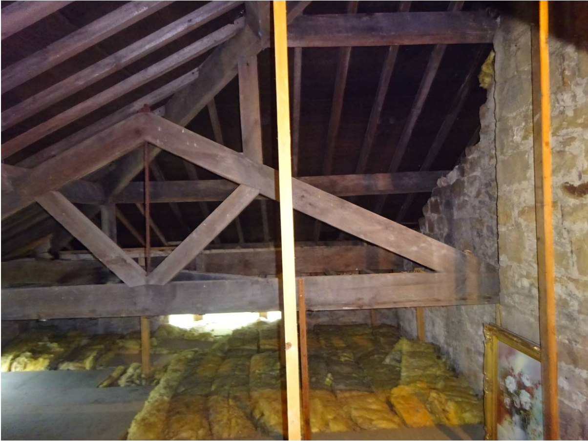
Roof Void – Original roof trusses / ceiling hangers
