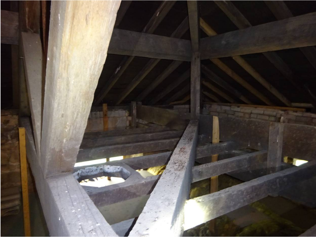
Roof Void – Original roof trusses / cross members / ceiling hangers
