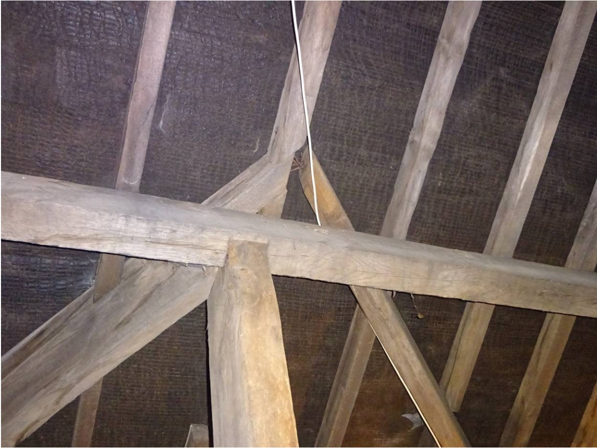
Rear Roof (over bedroom) – Open joint
