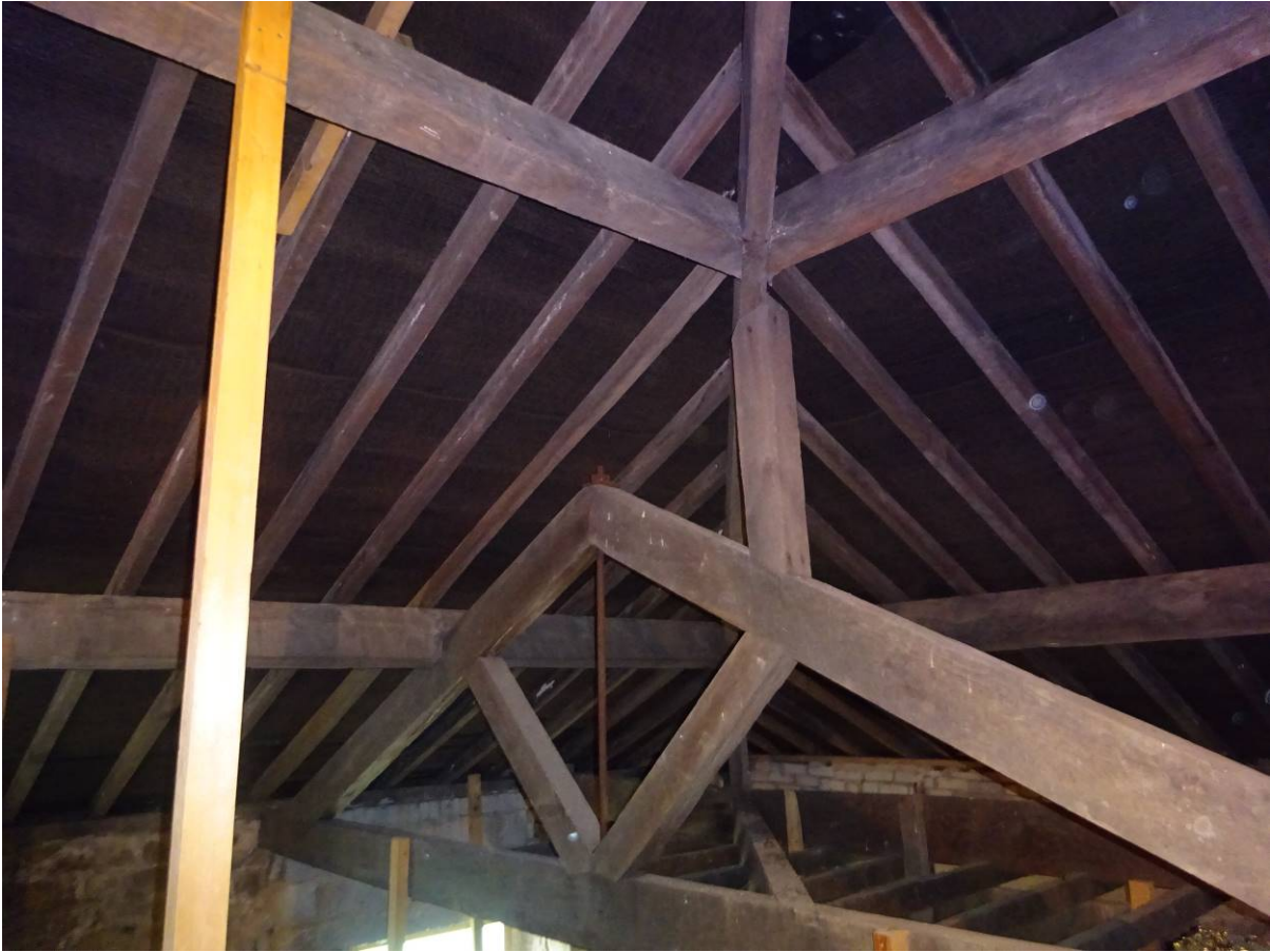
Roof Void – Original roof trusses / ceiling hangers
