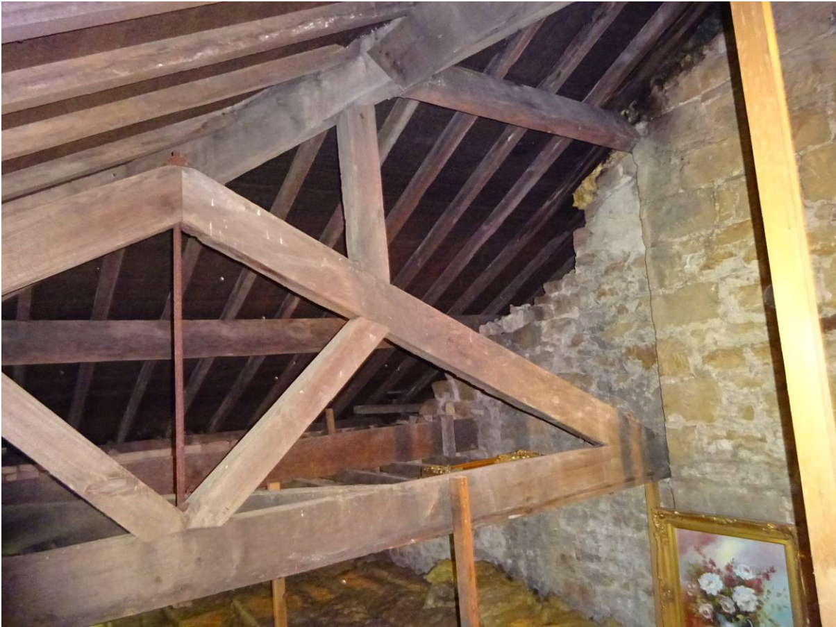
Roof Void – Original roof trusses / ceiling hangers
