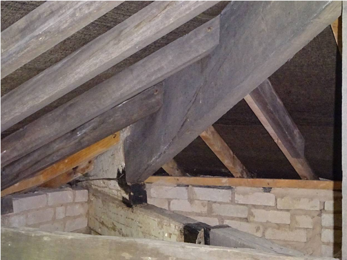
Rear Roof (over bedroom) – Open joint
