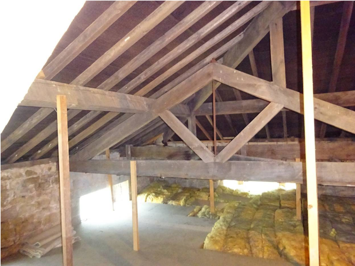
Roof Void – Original roof trusses / ceiling hangers
