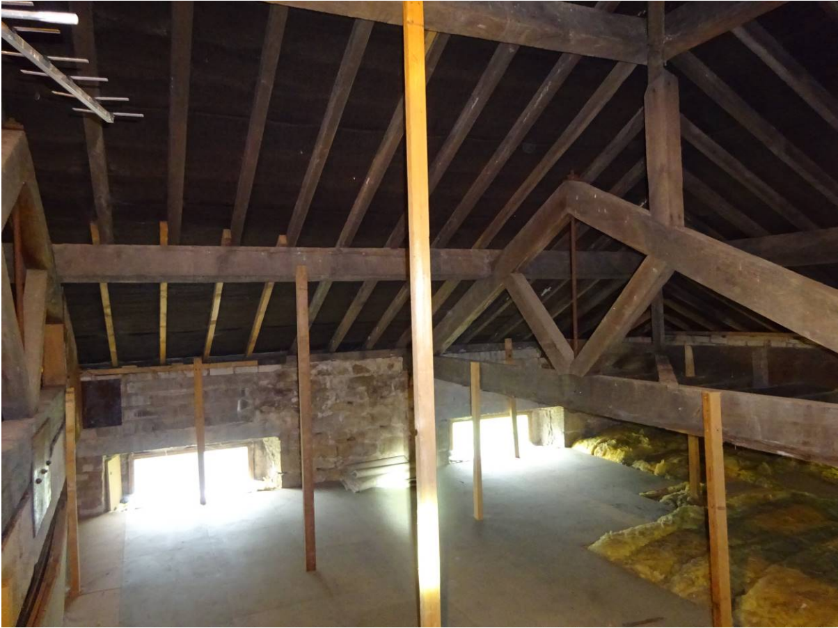
Roof Void – Original roof trusses / steel plates / original & replaced rafters / ceiling hangers
