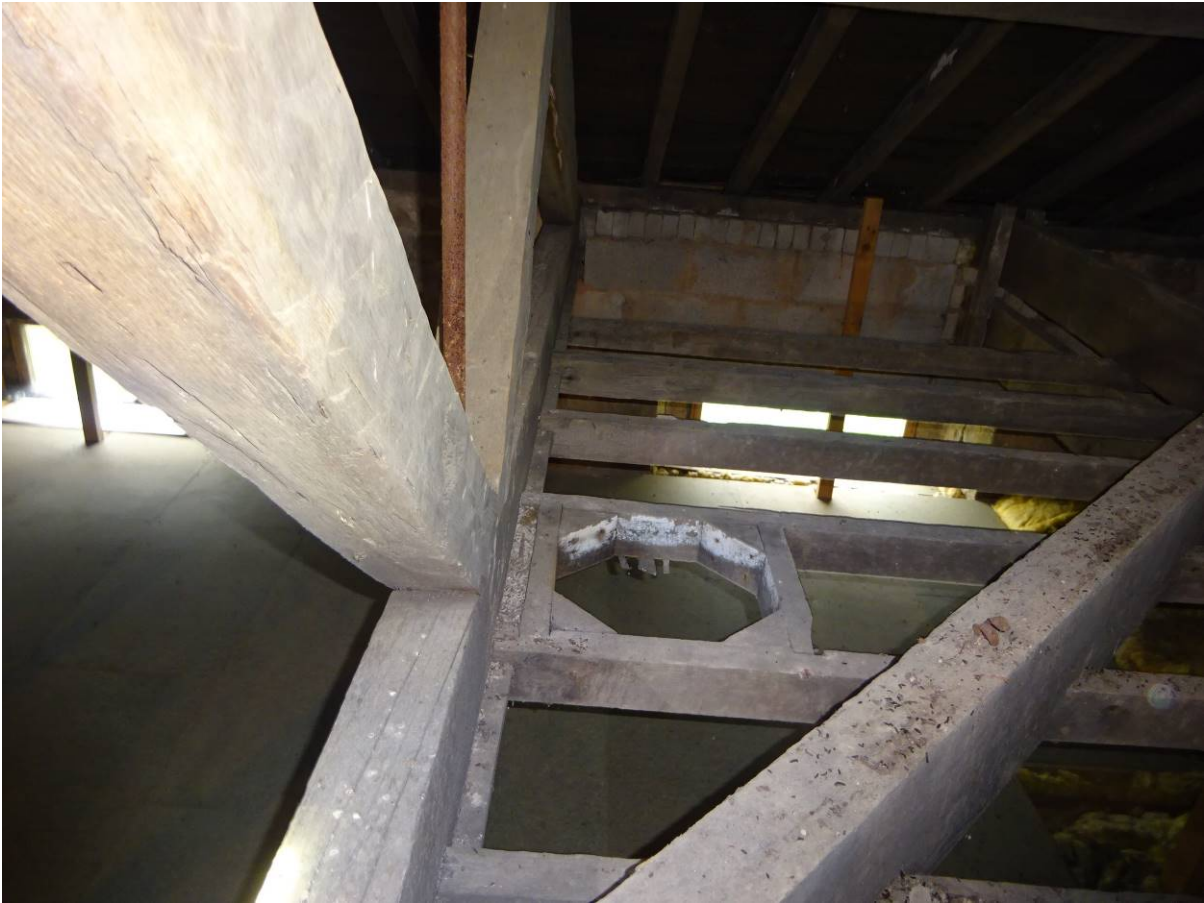
Roof Void – Original roof trusses / cross members / ceiling hangers
