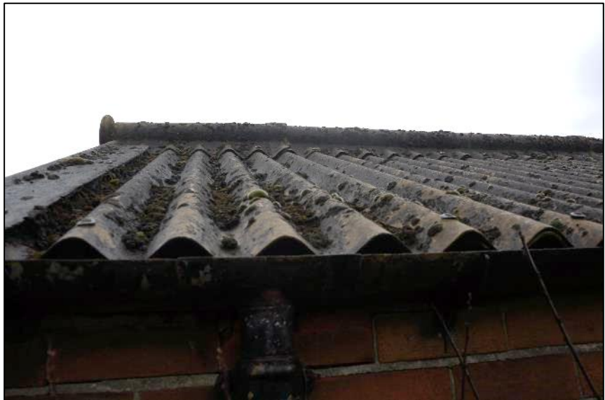
Photo 3: Corrugated asbestos roof sheets and metal guttering.
