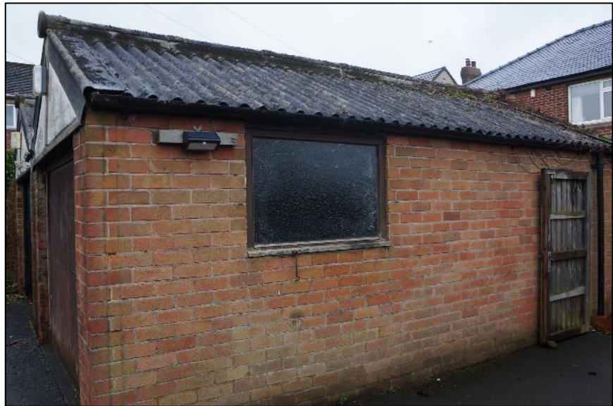
Photo 2: Northeast elevation with timber framed window, and fascia boards.
