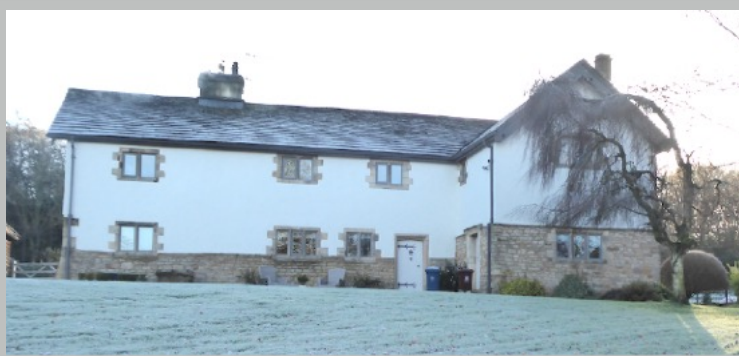
Plate 18. NW (river-facing) elevation of Dinckley Hall
