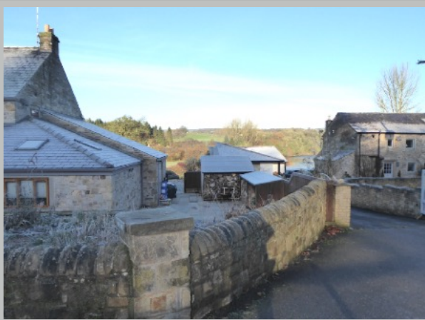
Plate 16. Existing outbuilding between Barn by the River and Ellis House
