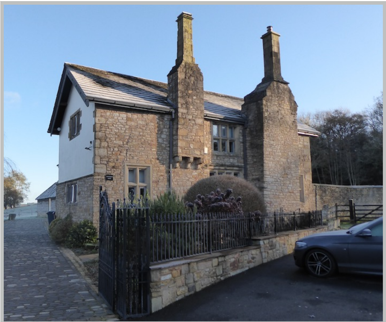
Plate 20. SW cross-wing and SE elevation of Dinckley Hall
