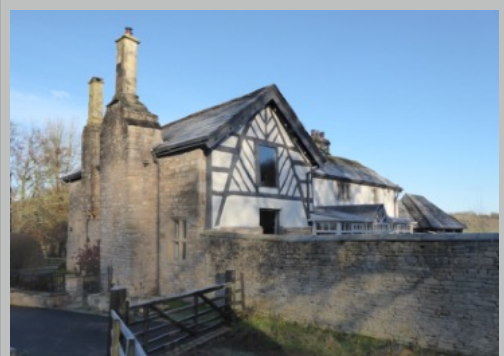
Plate 19. SW cross-wing and SE elevation of Dinckley Hall
