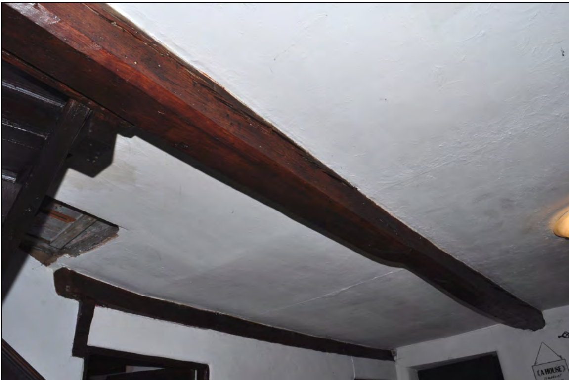
Photo 12: Beam 2, middle of lounge/living room (before work). Looking east.
