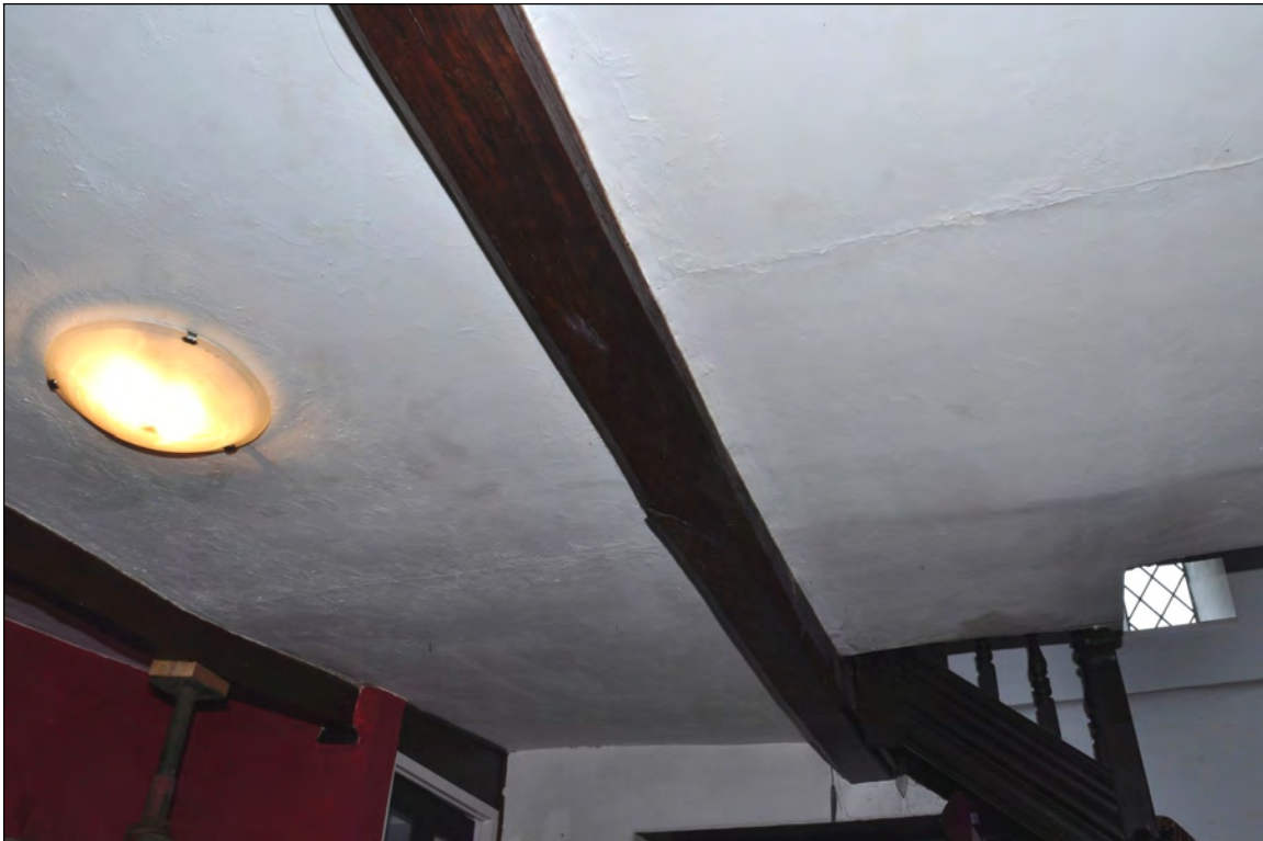
Photo 13: Beam 2, middle of lounge/living room (before work). Looking west.
