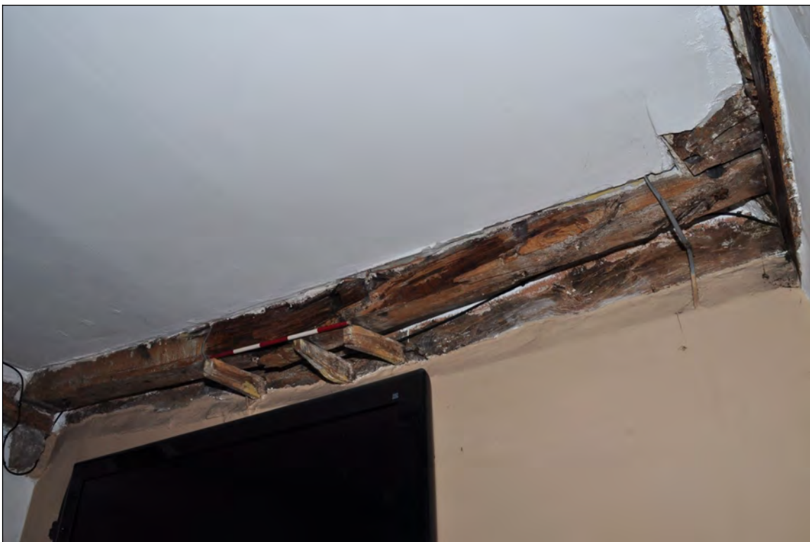
Photo 28: Beams 3 & 4, dining room (before work) . Looking south.
