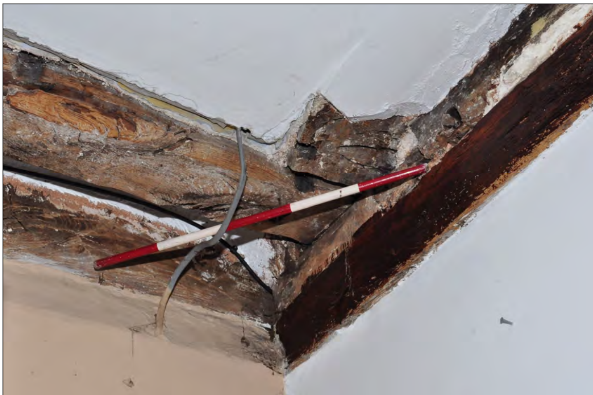
Photo 30: Beams 3 & 4, in dining room corner (before work). Looking west.
