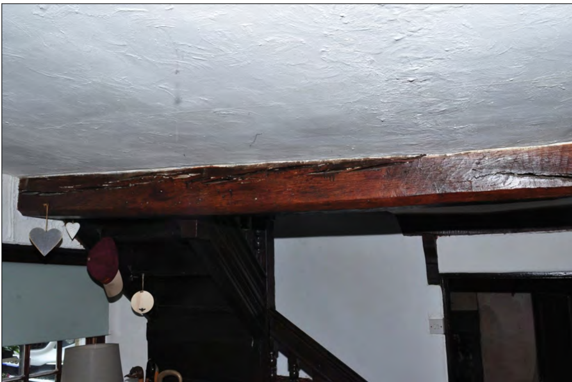
Photo 14: Beam 2, middle of lounge/living room (before work). Looking north-east.
