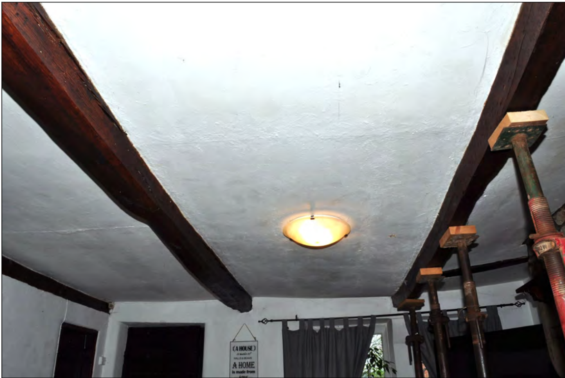
Photo 11: Beams 1 (right) and 2 (left), in lounge/living room (before work). Looking south-east.
