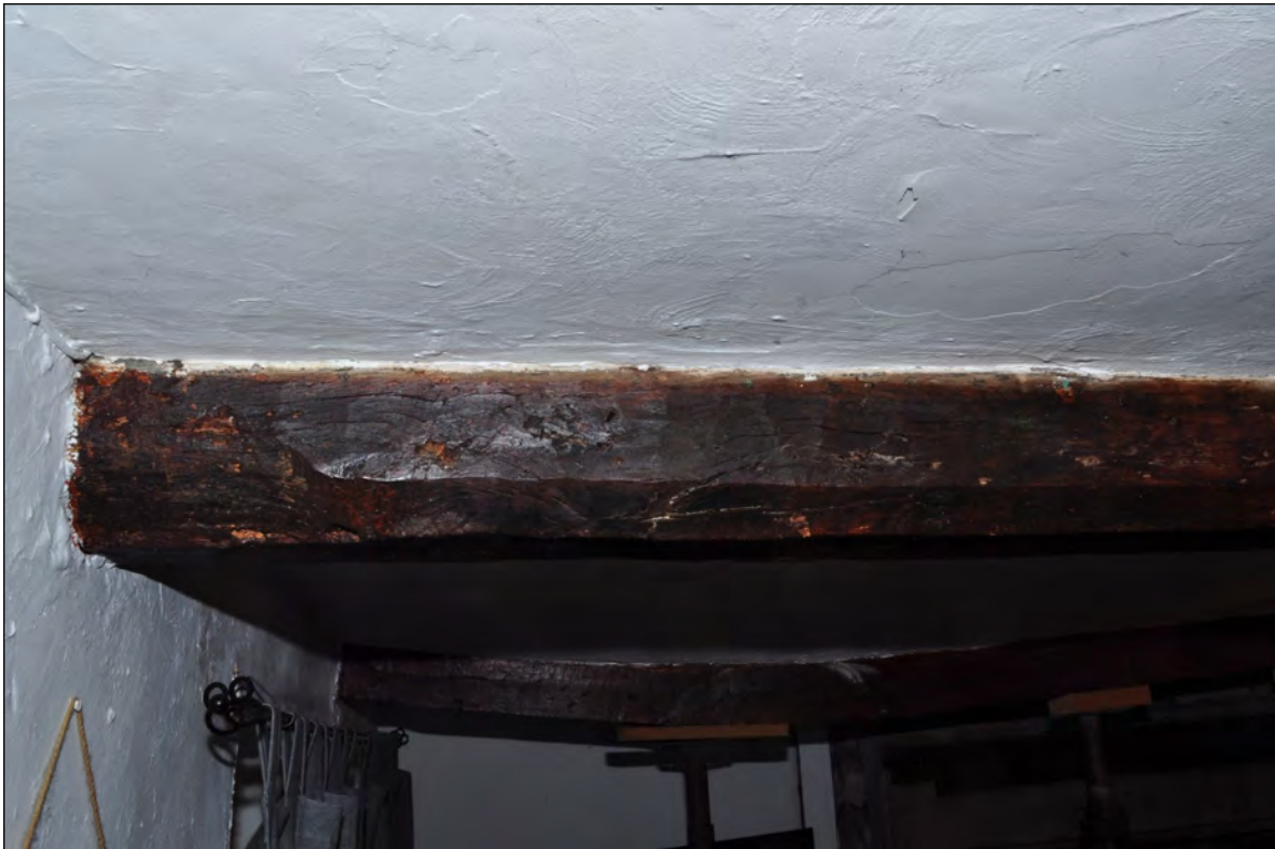
Photo 15: Beam 2, middle of lounge/living room (before work). Looking south-west.
