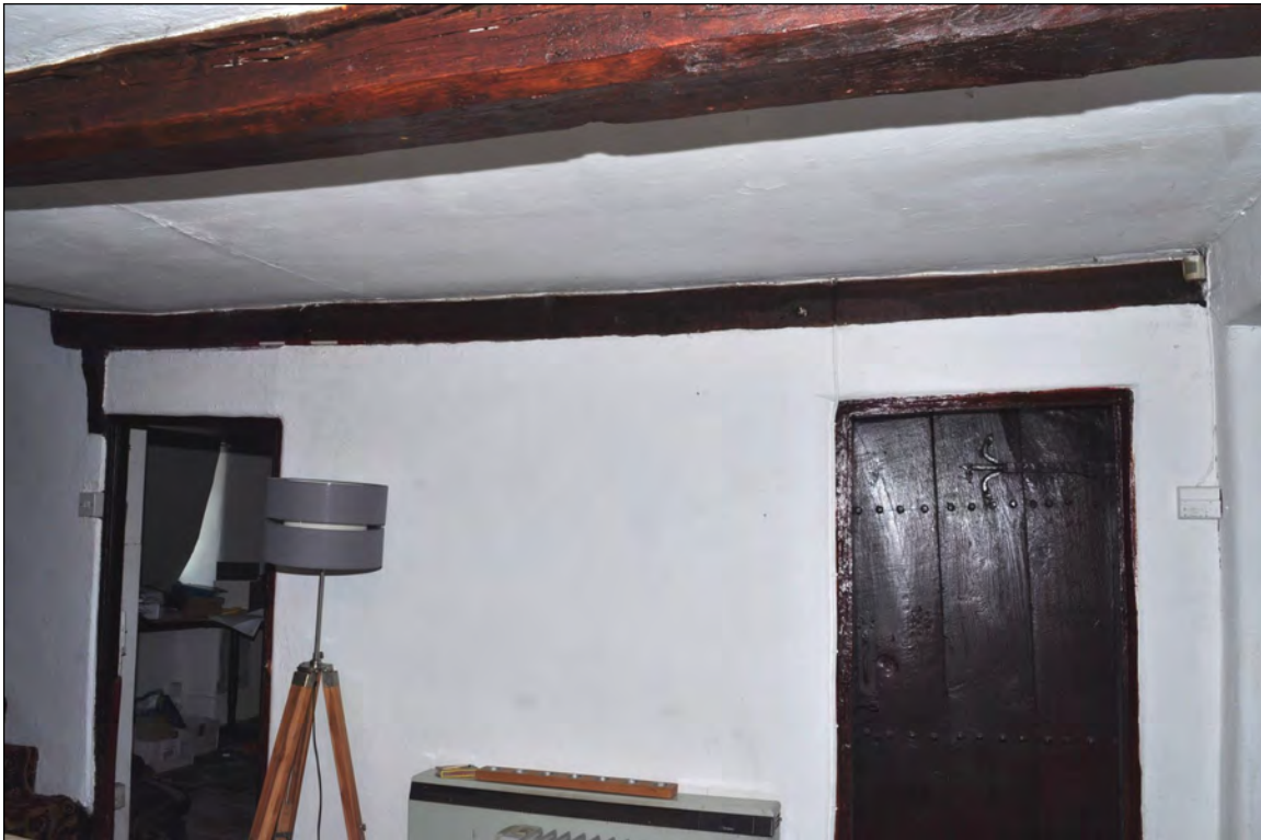
Photo 23: Beam 3 over partition between lounge/living room and study/dining room. Looking north.
