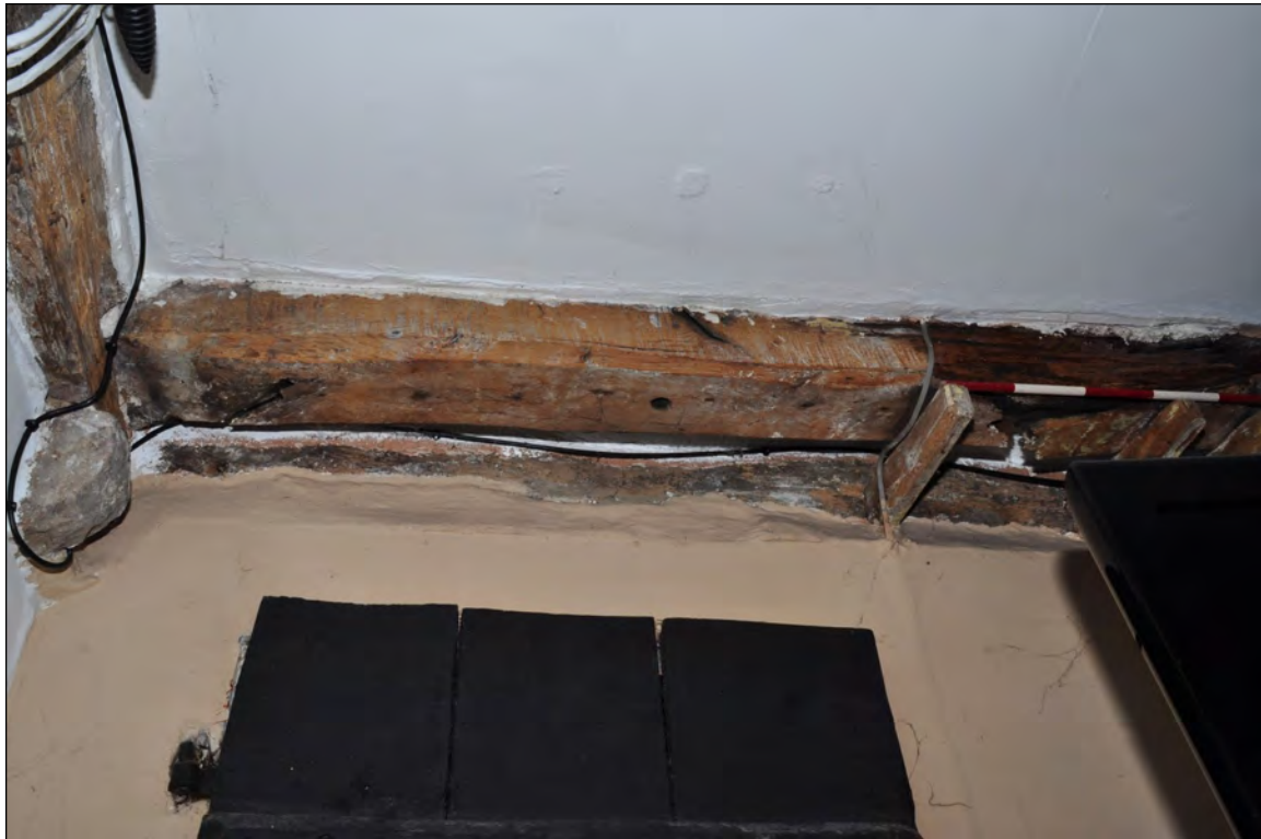
Photo 29: Beams 3 & 4, dining room (before work). Looking south-west.
