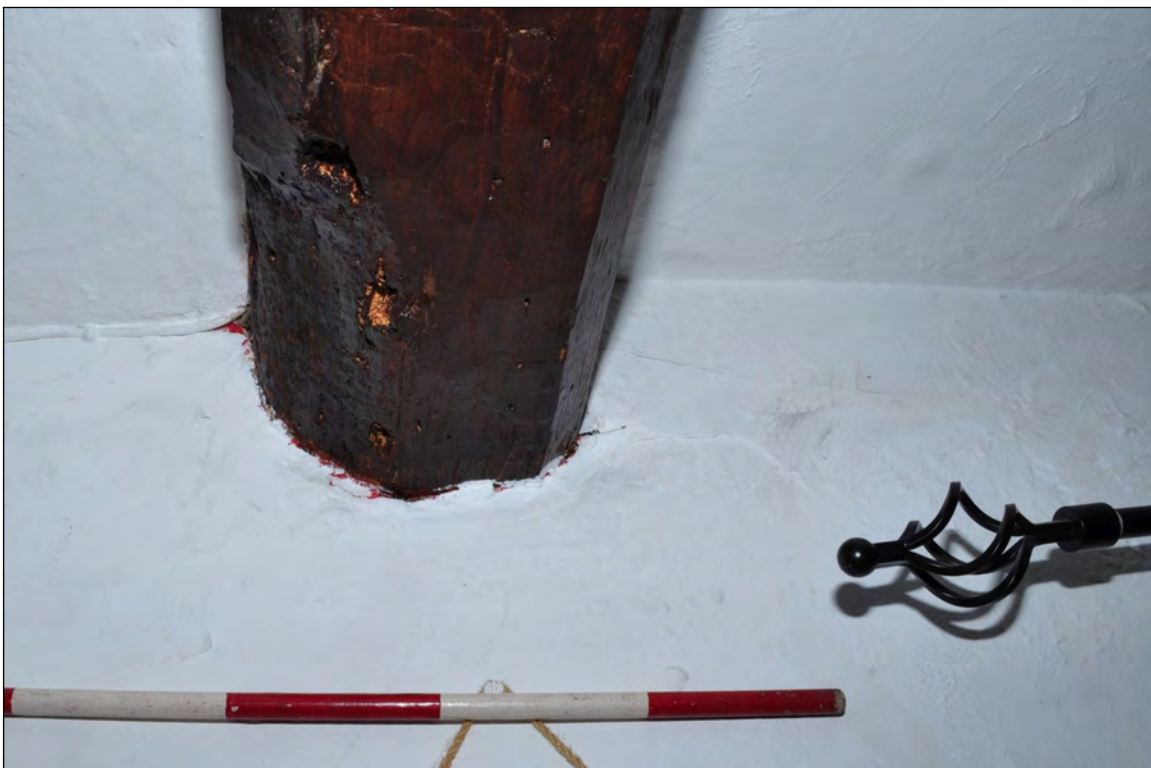
Photo 16: Beam 2, middle of lounge/living room (before work). Looking south-east.
