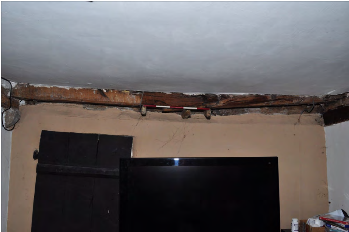
Photo 27: Beams 3 & 4, dining room (before work). Looking south-west.
