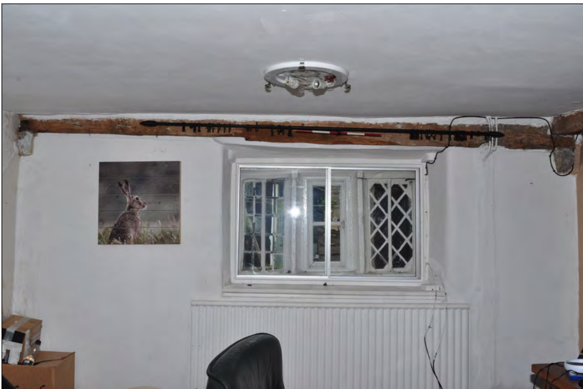
Photo 34: Beam 6, by outer wall of dining room (before work). Looking south-east.
