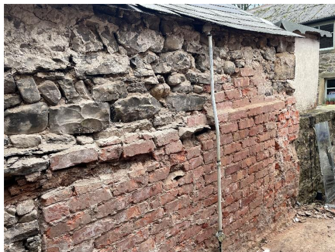
Figure 2 – Alternative view of exposed wall.
