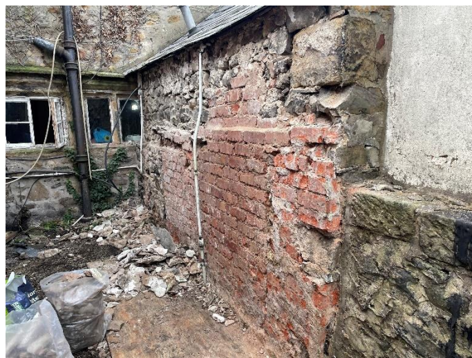
Figure 1 – View of exposed wall.
