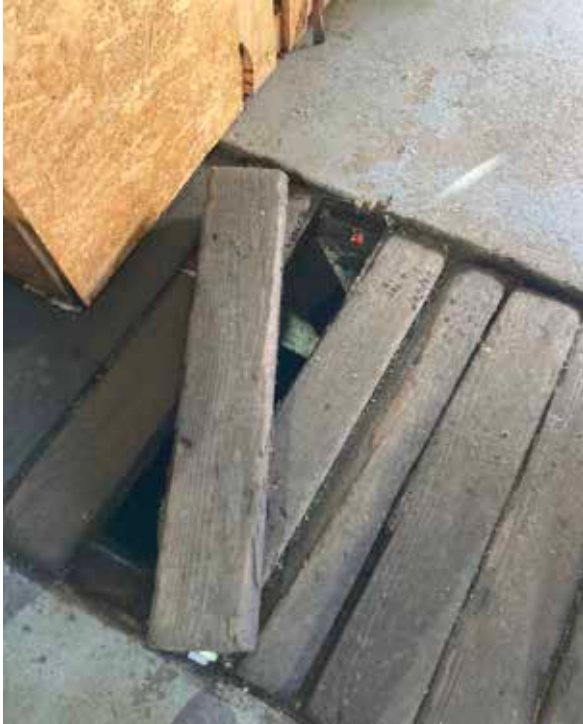
Photo 9: Timber cover to vehicle inspection pit.
