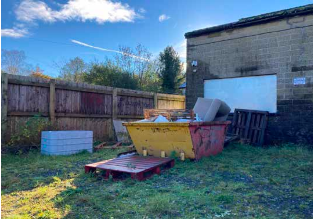
Photo 7: Waste skip and pallets next to north-east corner of garage building.
