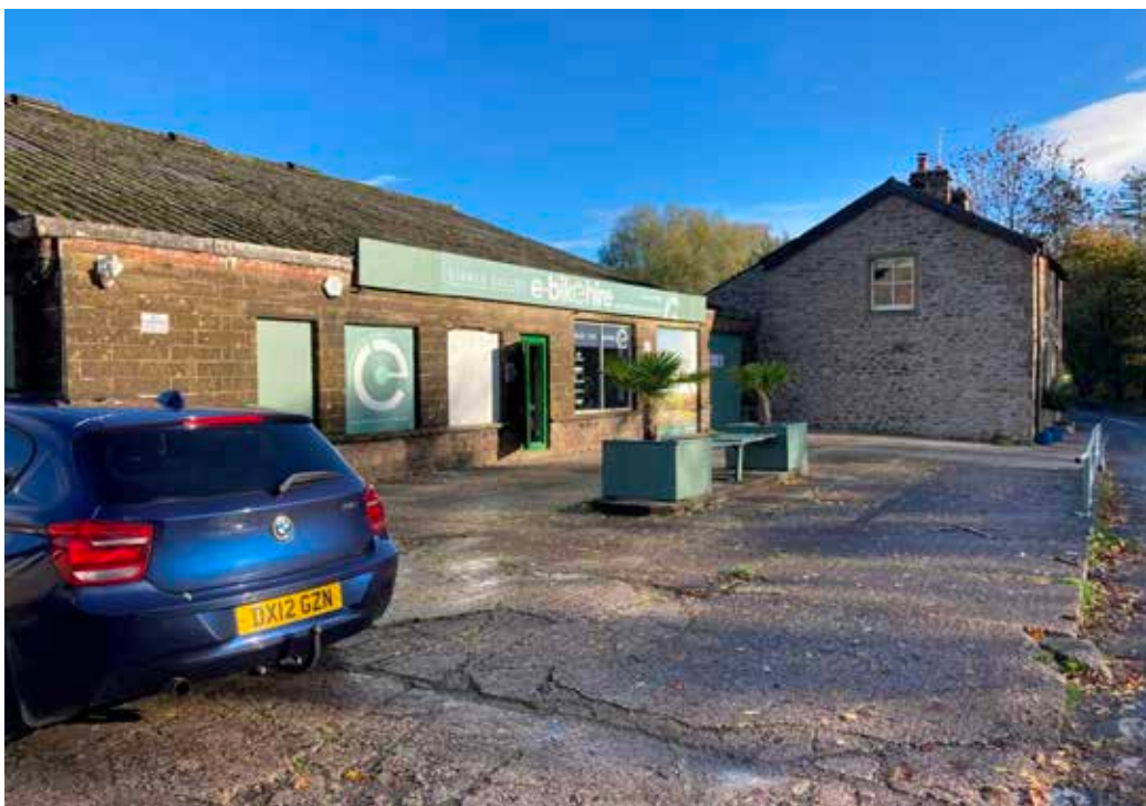
Photo 2: View looking eastwards across former petrol filling station forecourt, with Forge House beyond.
