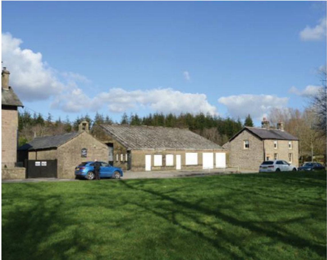
Figure 5: Existing garage site (Source: Google Earth).
