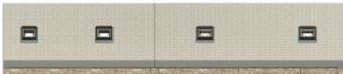
Roof Lights rear elevation
