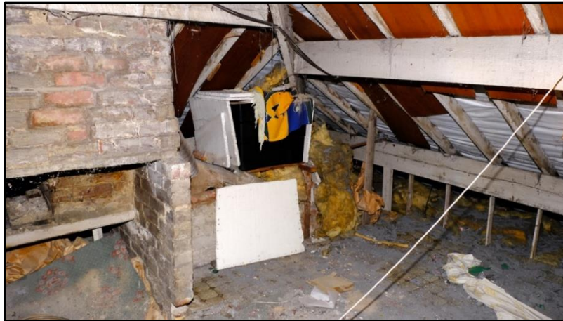
Internal view of roof void showing brick chimney, modern roof liner and wood panel underboarding the roof structure
