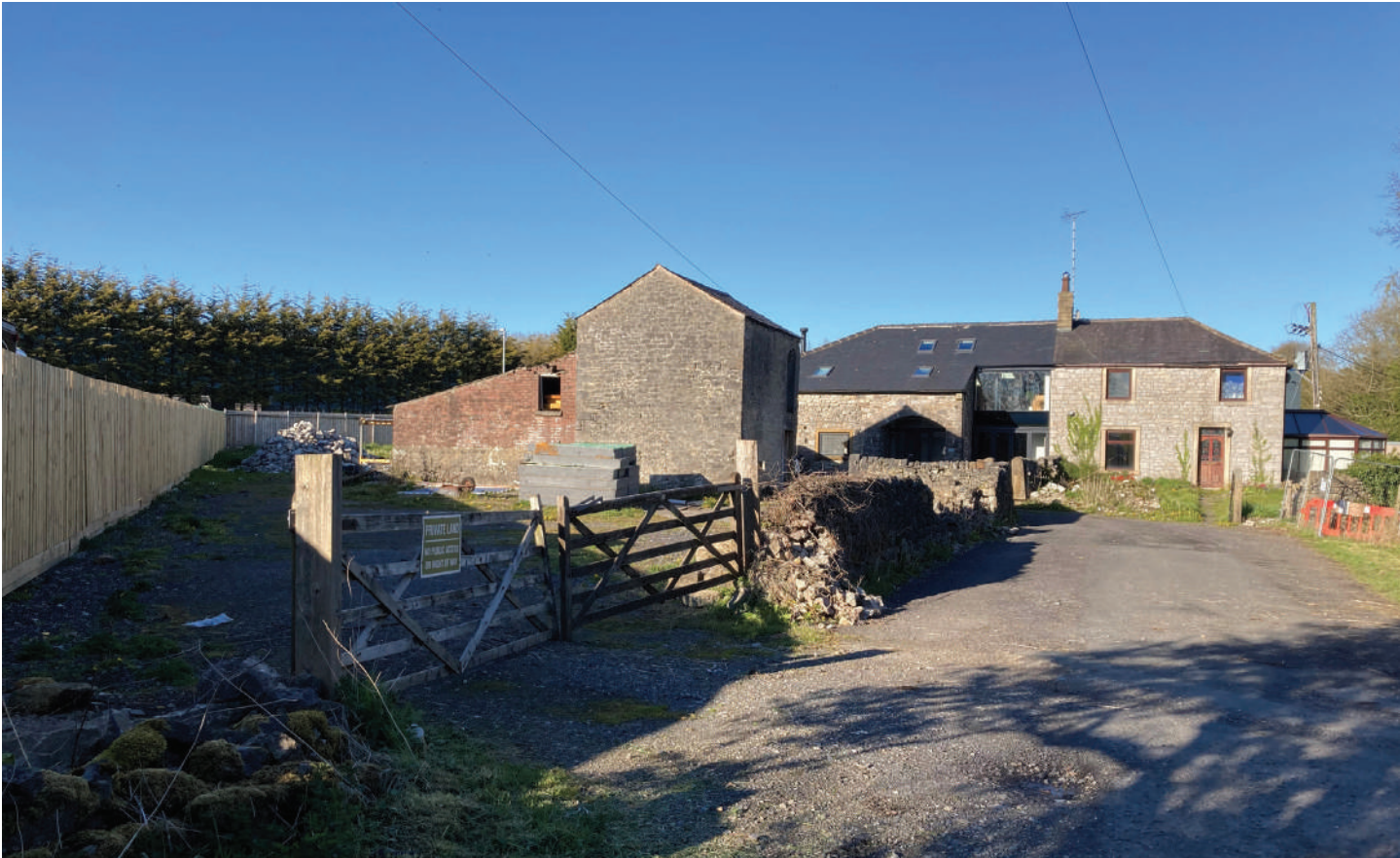
PL05: Photograph of the existing site entrance
