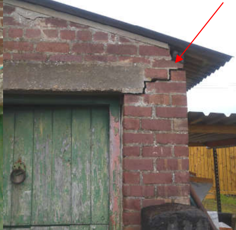
Photo (4)- north east corner of lean -to
