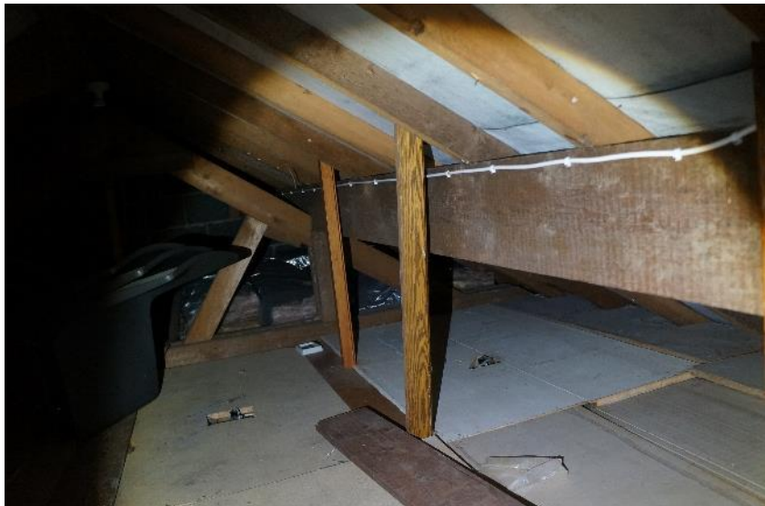
Photo 7: Internal view of the loft space showing roof lining and timber beams.
