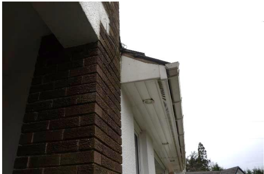
Photo 5: uPVC soffits and guttering on front (west) elevation..
