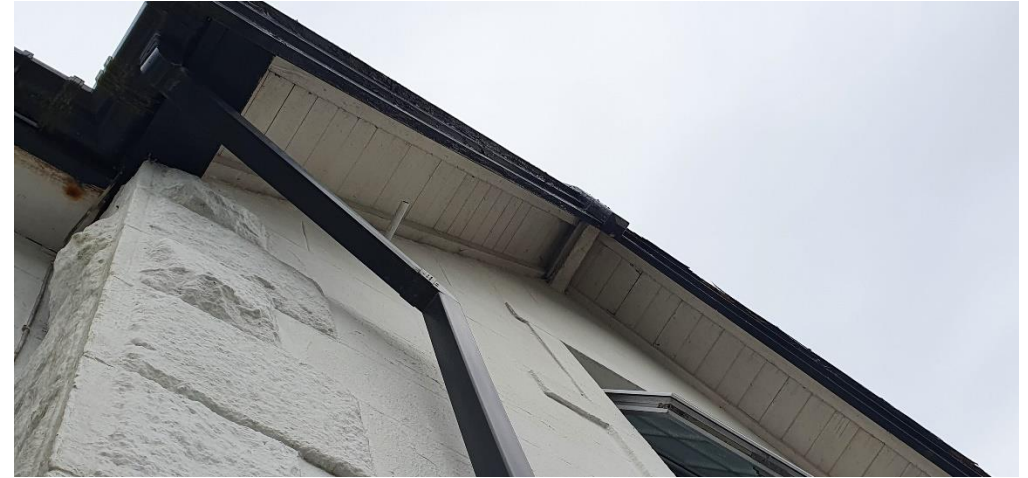
B1 – wooden soffits present along the eastern gable (pictured above).
