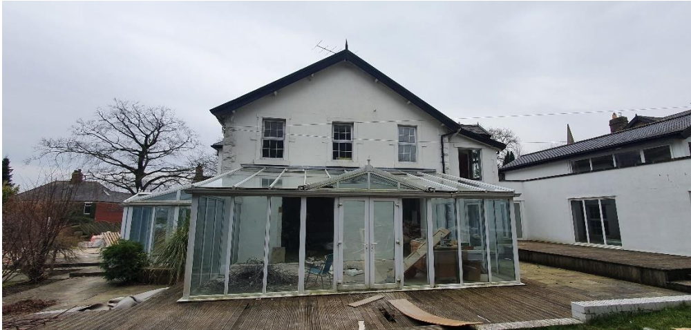
B1 – northern elevation (pictured above).
