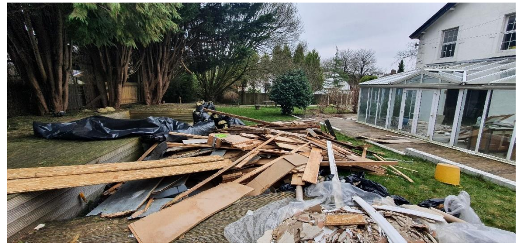
B1 – internal ceilings and roof insulation removed from B1 (pictured above).
