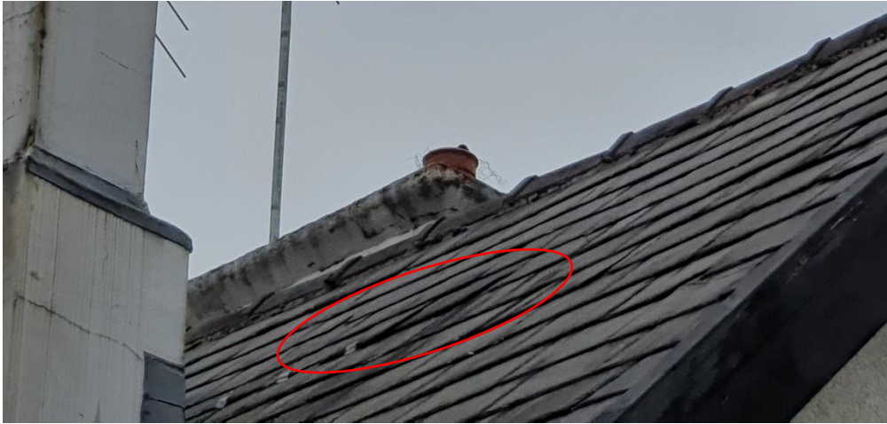
B1 – southern elevation roof and lifted tiles as pre the previous ecological report (pictured above).
